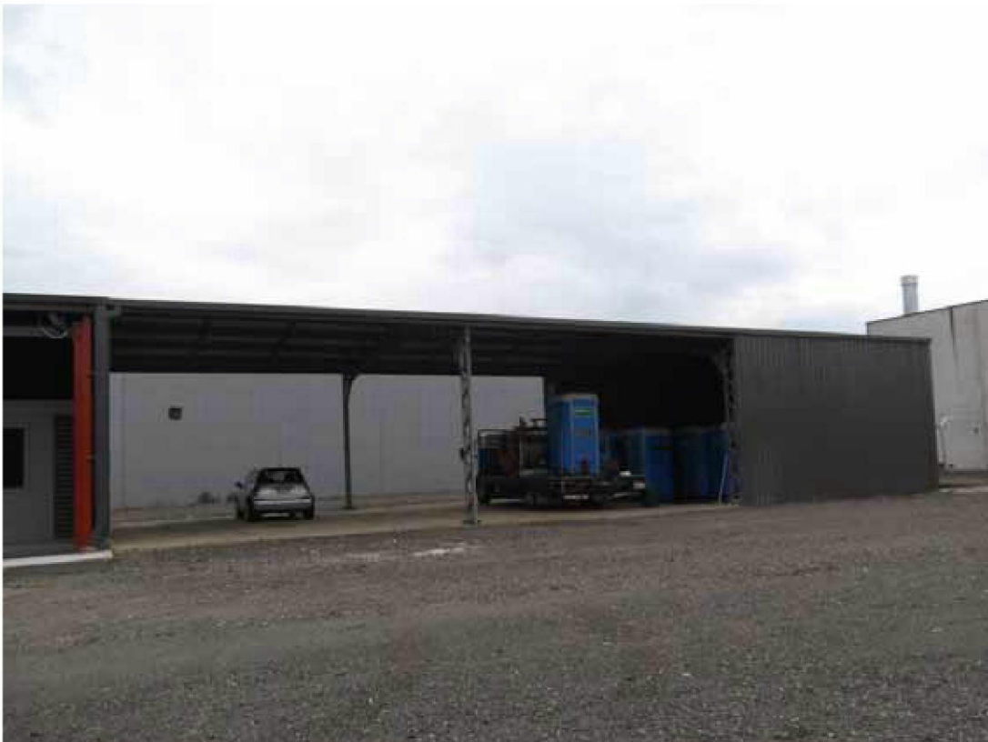
Photo 6: View of existing structure
