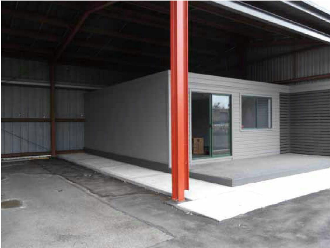
Photo 7: View of office in existing structure
