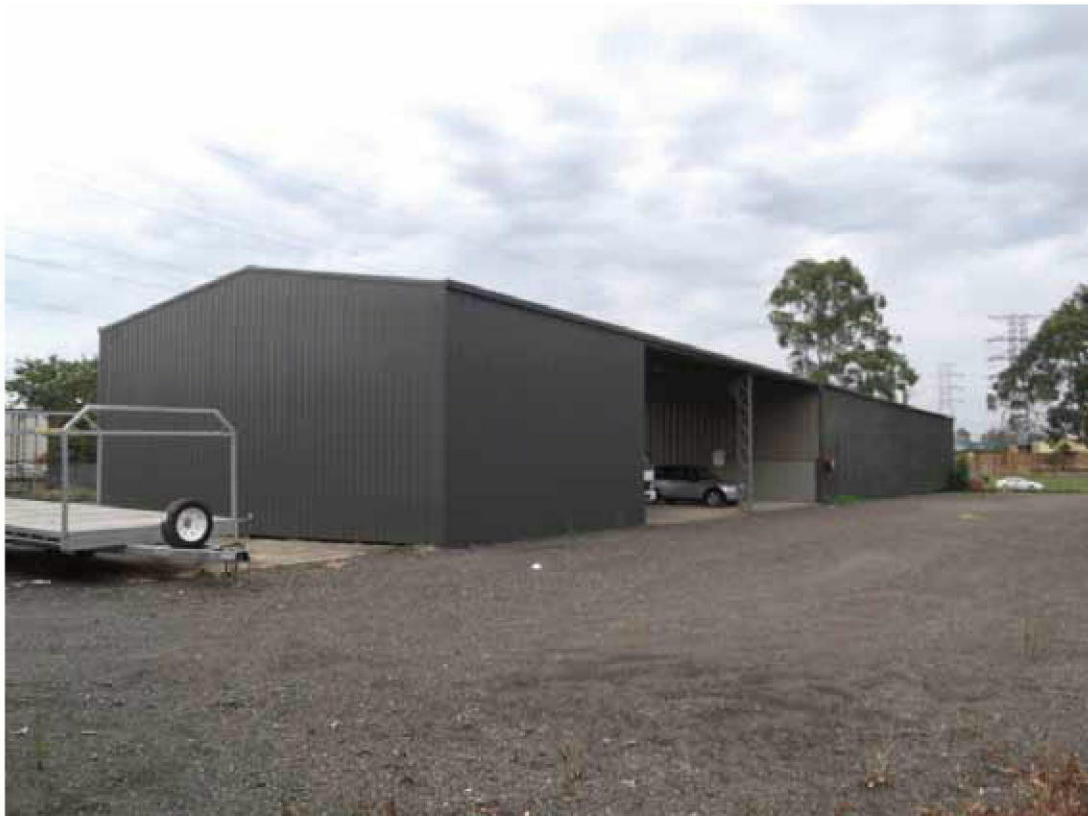
Photo 4: View of existing structure from South West corner
