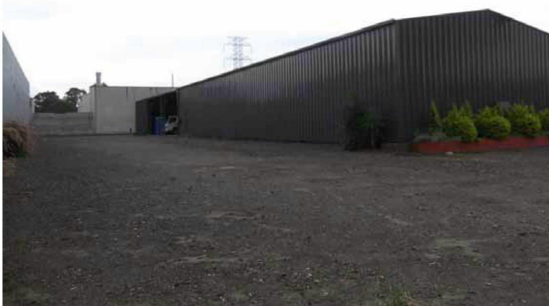
Photo 3: View of existing structure from South East corner
