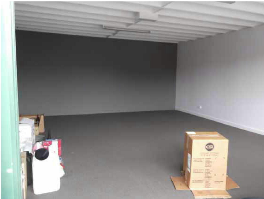
Photo 8: View inside office
