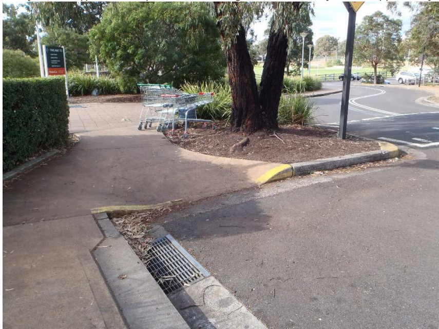
Figure 6 Photo of T2, Eucalyptus sideroxylon . The photo shows the location of the stormwater inlet pit, and the exposed surface roots, pram ramp and garden bed extent which is proposed to remain with TPZ fencing to protect.
