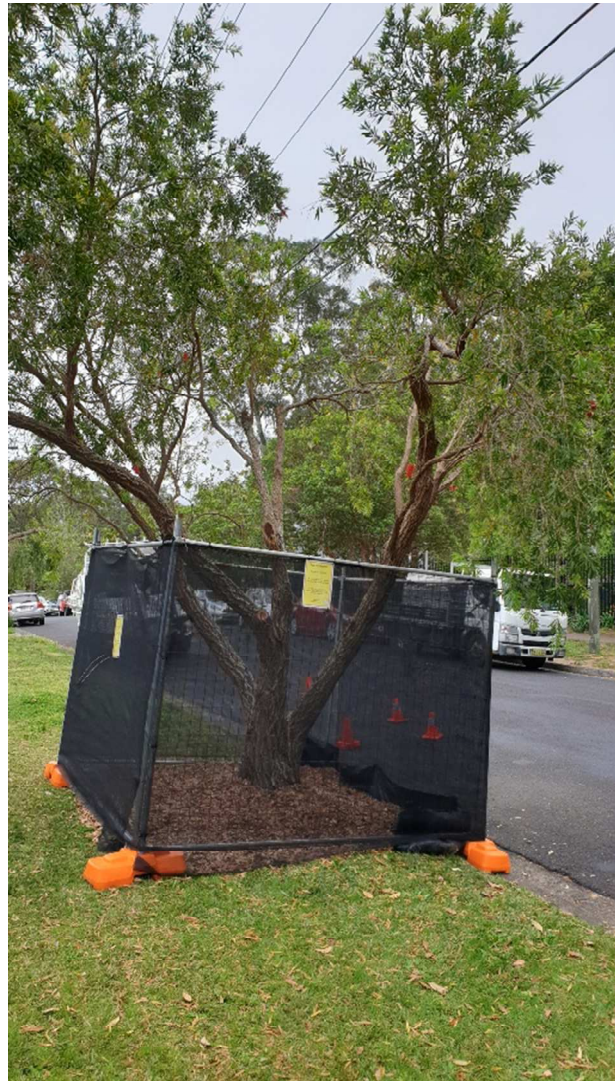
Figure 4. Example of tree protection fencing and signage..
