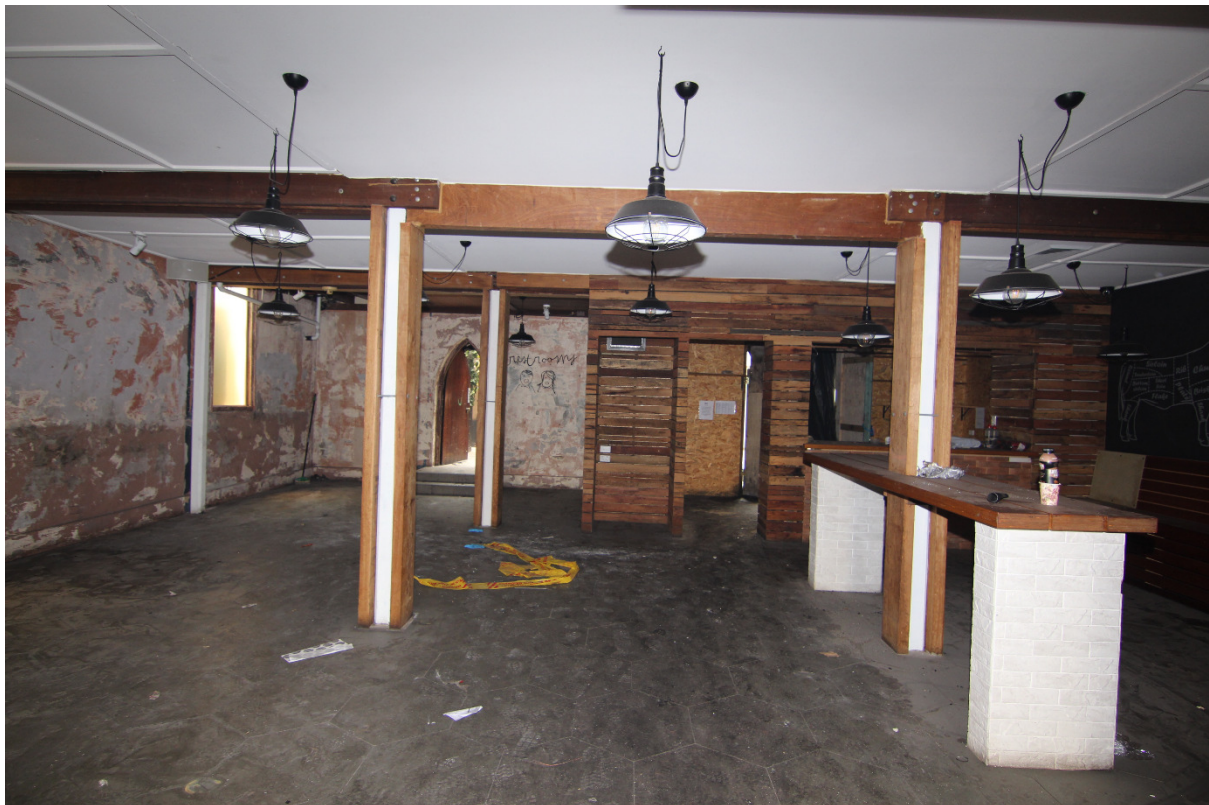
Fig. 14: View of ground floor restaurant area – note the columns supporting first floor loft area. (Source: Steven Guadagnin, November 2019.)
