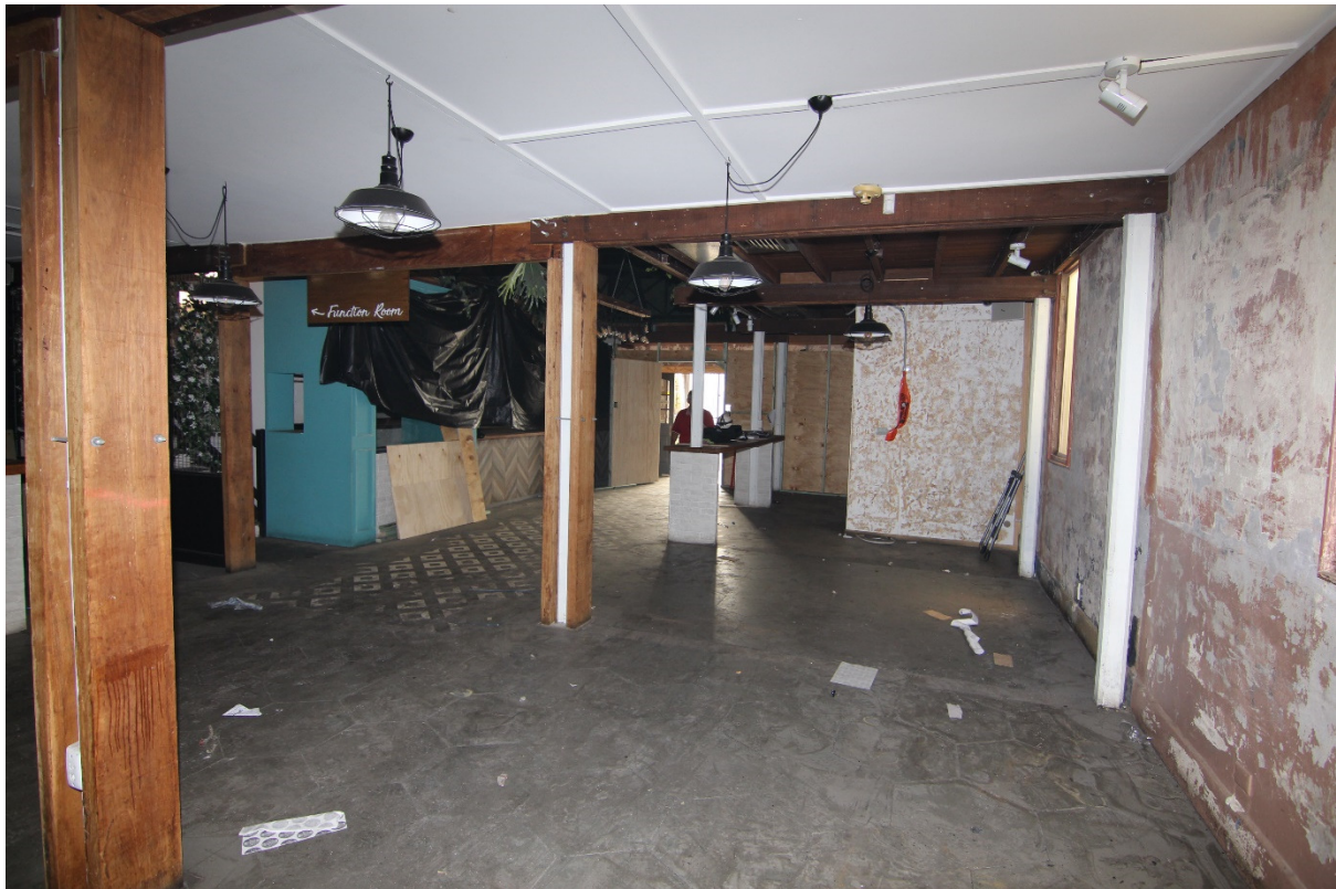
Fig. 13: View of ground floor restaurant area – note the columns supporting first floor loft area. (Source: Steven Guadagnin, November 2019.)
