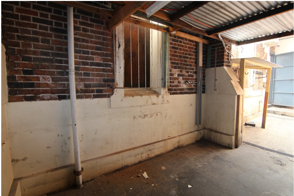
Fig. 9: View of rising damp affecting brickwork and render along west elevation. (Source: Steven Guadagnin, November 2019.)
