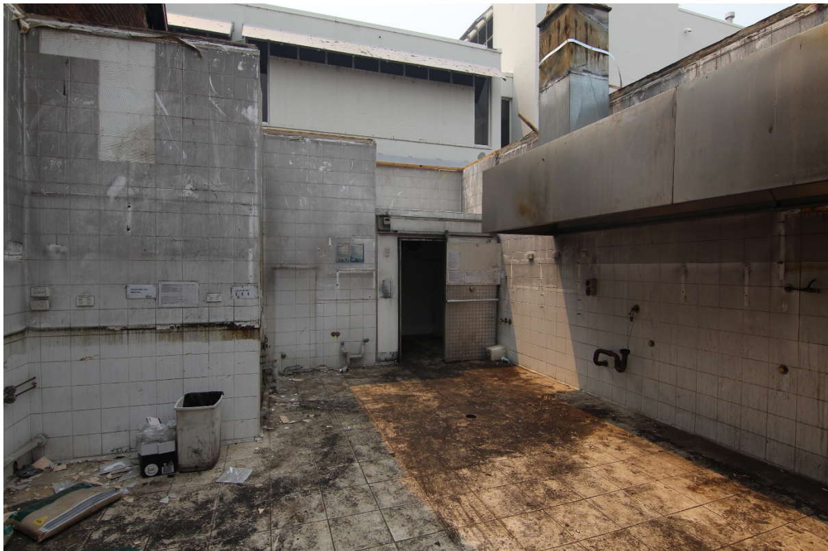
Fig. 16: View of kitchen area – note the roof above kitchen area demolished as part of make safe works. (Source: Steven Guadagnin, November 2019.)
