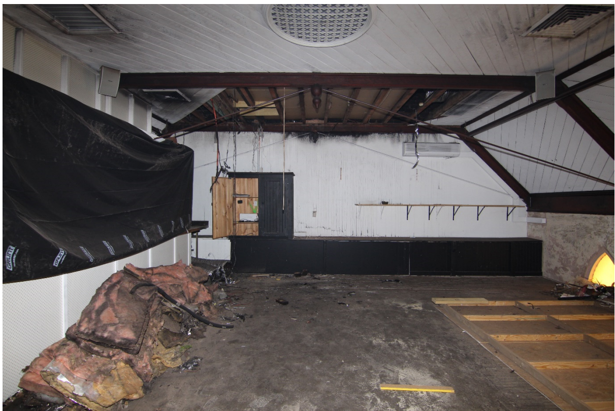
Fig. 18: View of first floor loft dining area – note the area of fire damaged roof. (Source: Steven Guadagnin, November 2019.)
