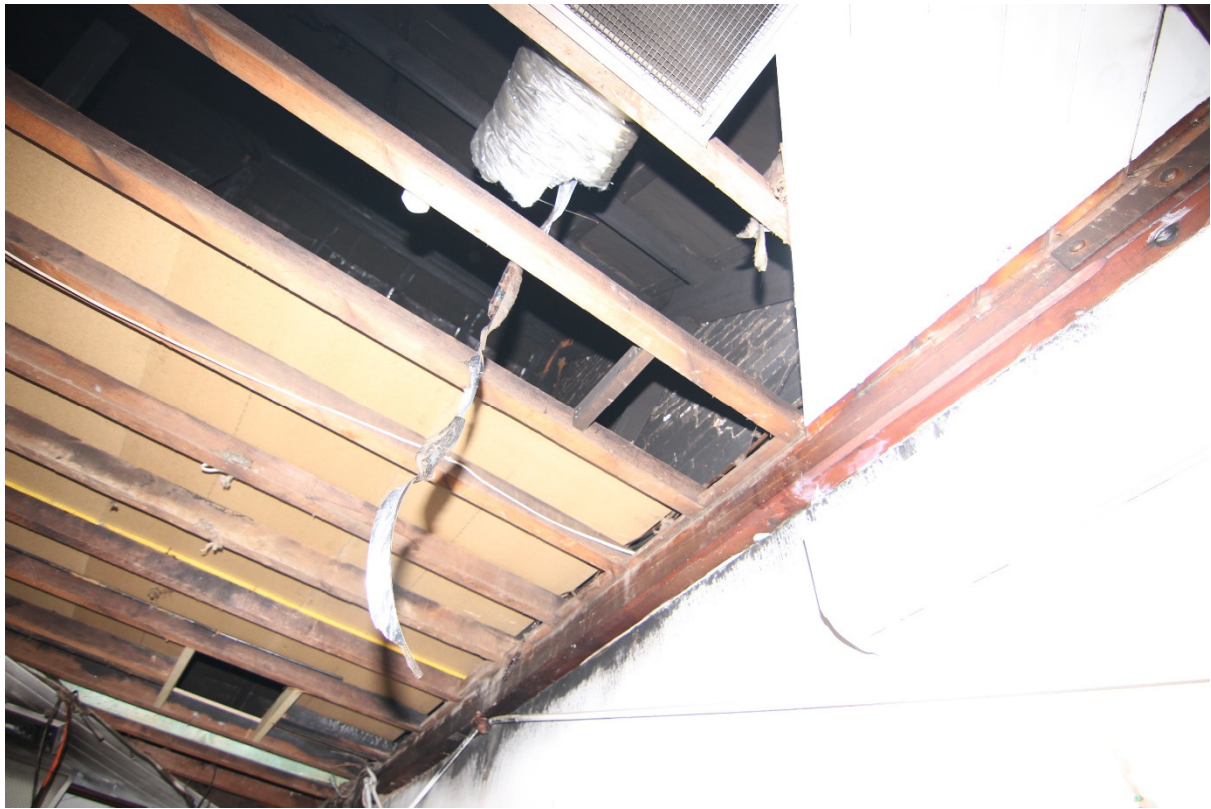
Fig. 19: View of fire damaged first floor roof framing. (Source: Steven Guadagnin, November 2019.)
