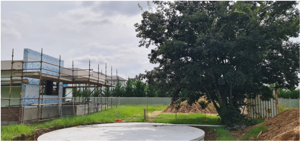
Further rear view of dwelling under construction and development site.
