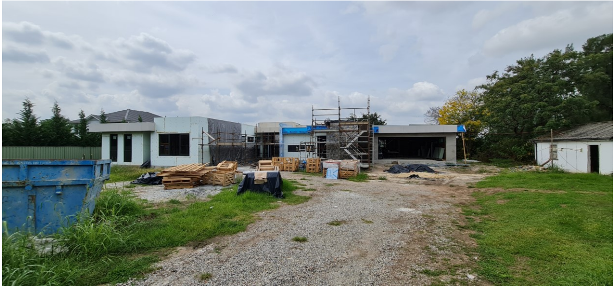
Further front view of site with dwelling under construction.
