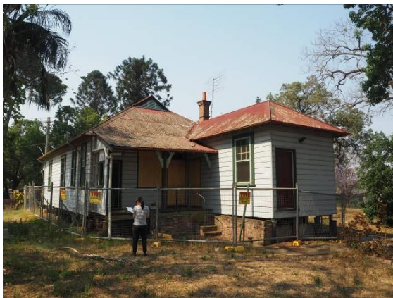
Figure 5: Southern (rear) elevation of the former Police Station and Residence.
