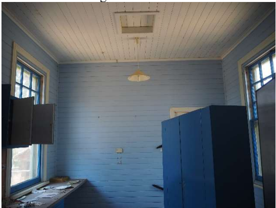
Figure 11: Interior view of existing kitchen looking south (room 8).
