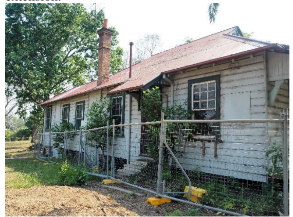
Figure 6: East elevation of the former Police Station and Residence, with original main entry.
