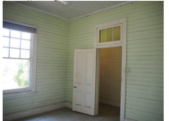
Figure 12: Interior view of existing bedroom (room 1), looking southeast.
