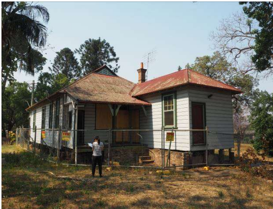
Figure 7: Southern (rear) elevation of former Police Station Building.
