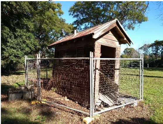
Figure 9: The original weatherboard double privy located in the rear garden of the allotment.
