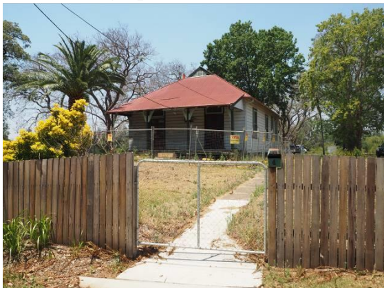
Figure 3: Front (north) elevation of the former Police Station and Residence.
