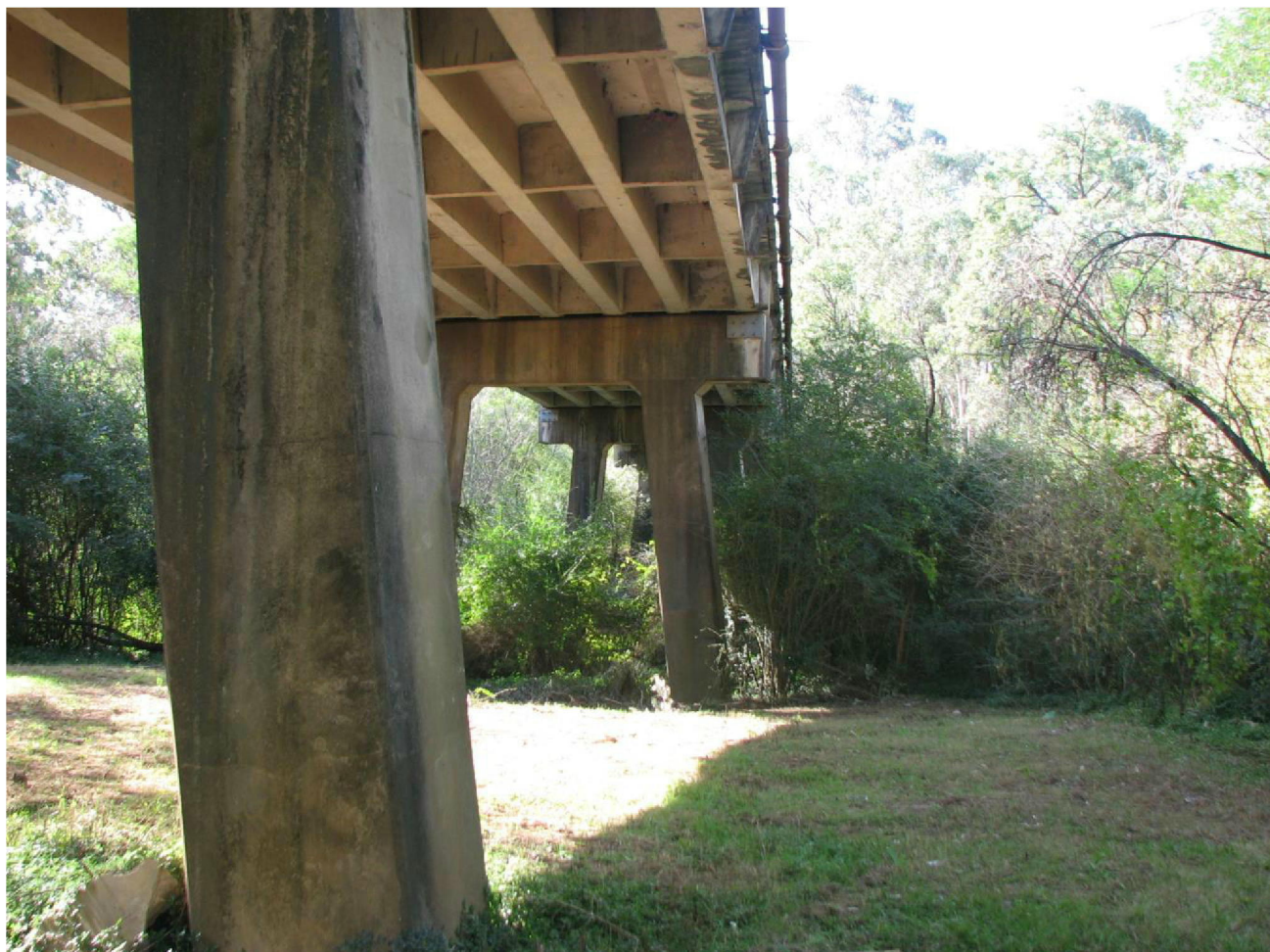
Figure 5 Existing South Creek Bridge
