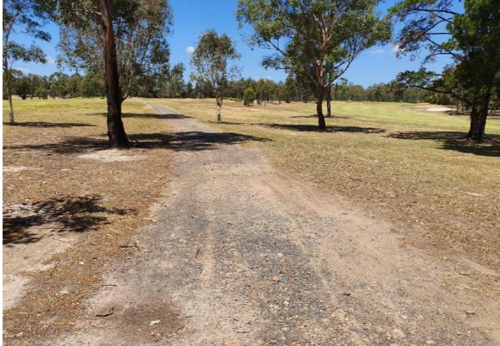
Photo 1 - Graded aggregate on the surface of an access way (facing east)
