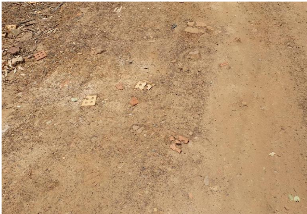
Photo 3 - Bricks and concrete observed adjacent to the potential ACM in the fill access way
