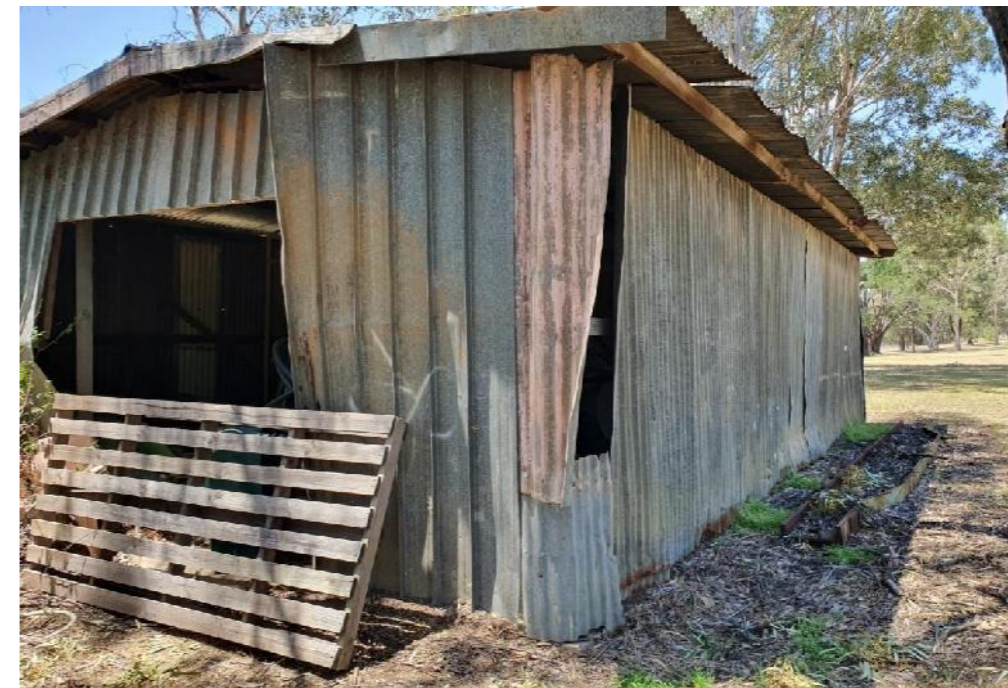
Photo 4 - Easternmost shed (facing east)
