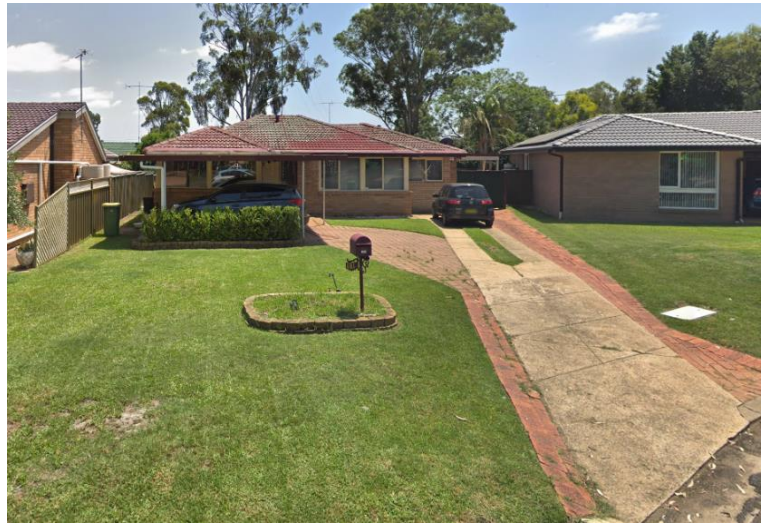
Street view of the subject site
