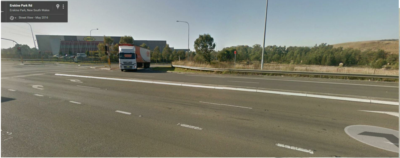
STREET VIEW FROM ERSKINE PARK ROAD
