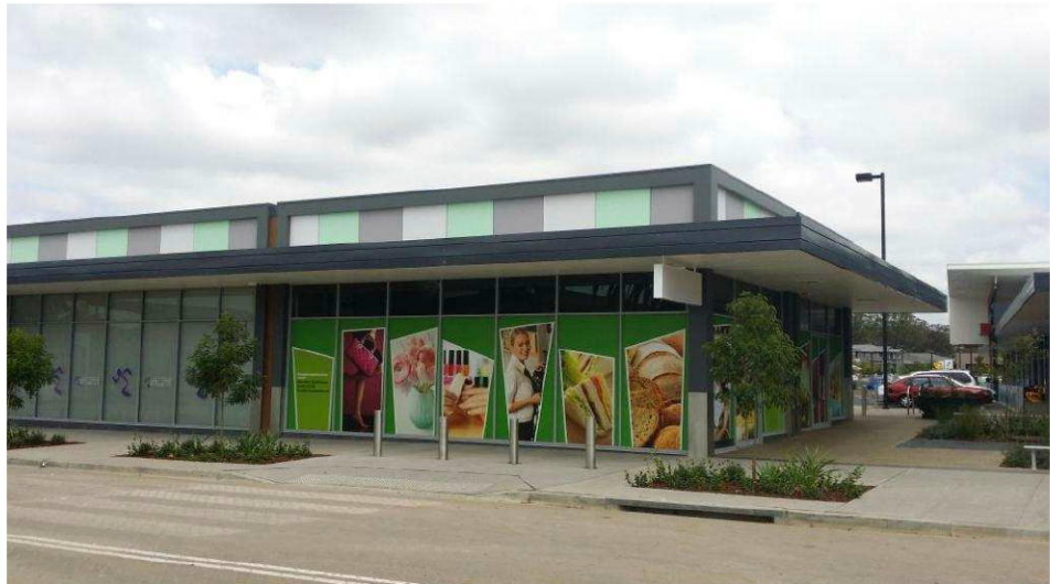
Figure 5 – View of shop premises to the south of the Woolworths car park, along Jordan Springs Boulevard
