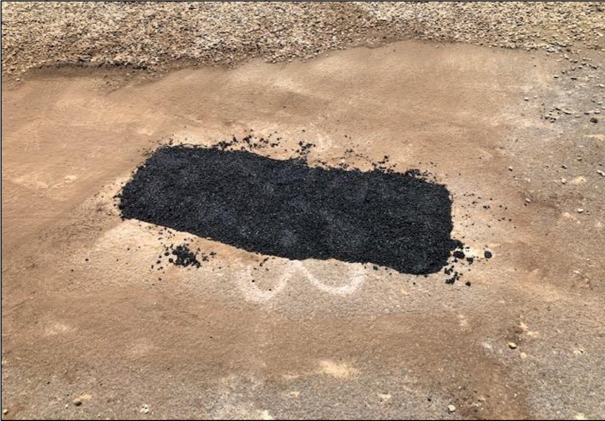
Photograph 3. Test Pit CC78 after being backfilled.
