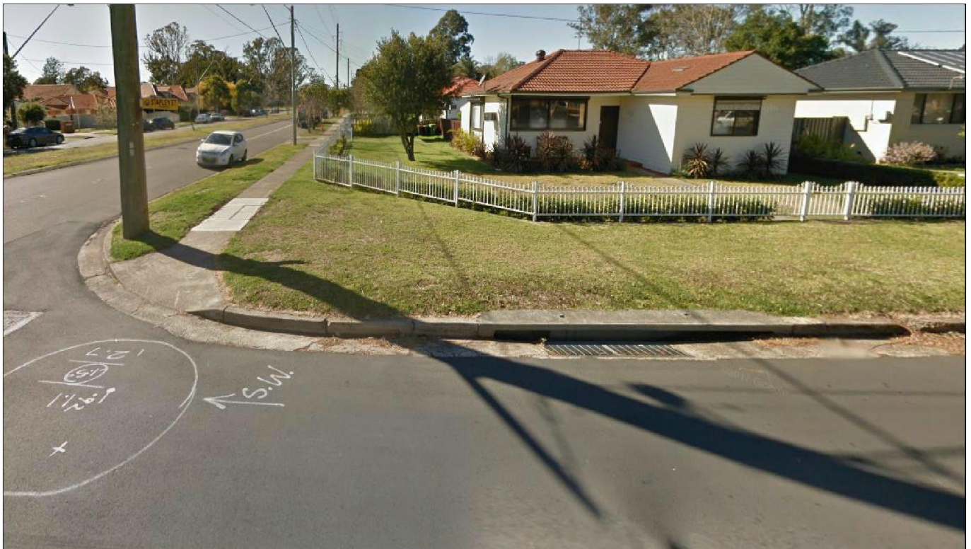
Figure 3 Existing kerb inlet pit at 36 Stapley Street, Kingswood (Downstream)
