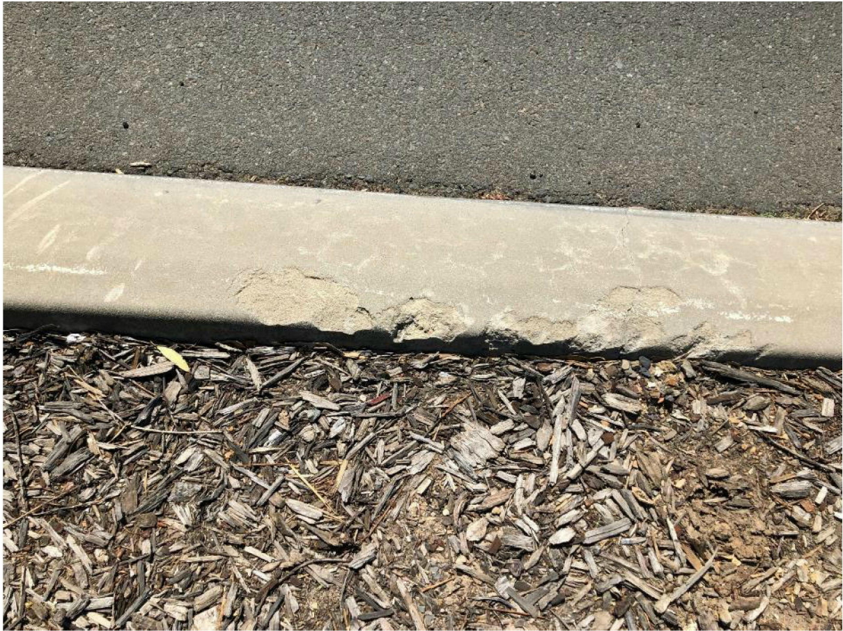
Figure 20: chips on top of median strip kerb.
