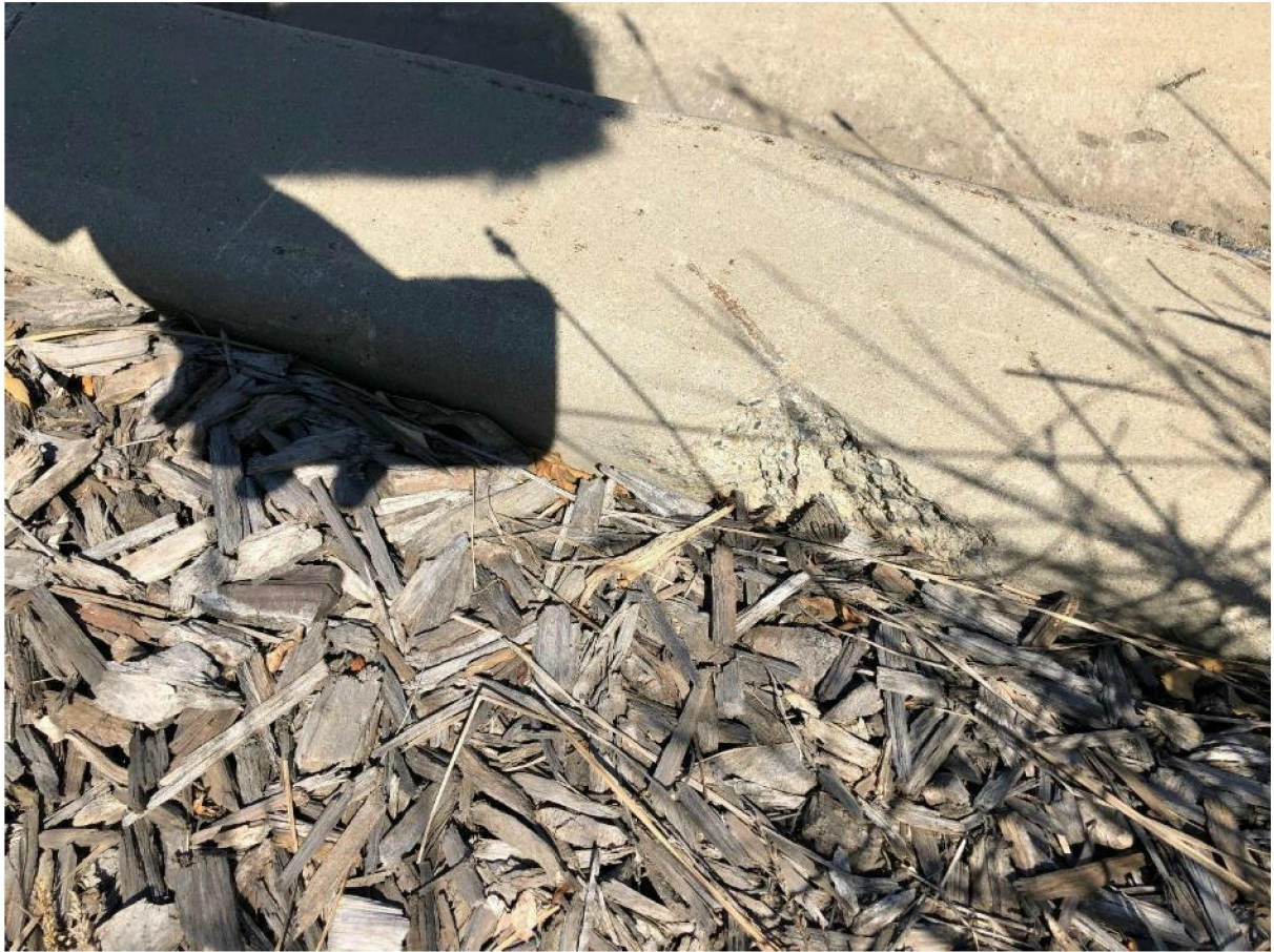
Figure 80: chip to top of kerb.
