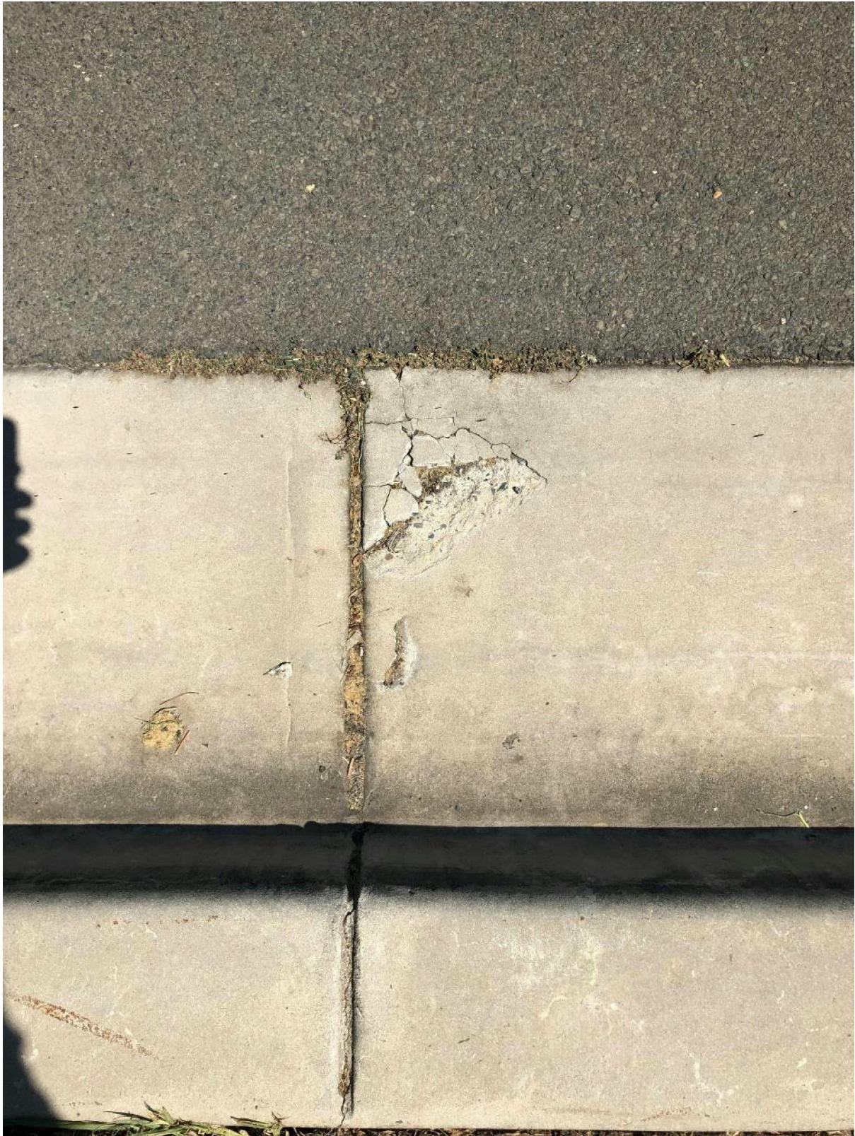
Figure 69: chip to gutter construction joint interface.
