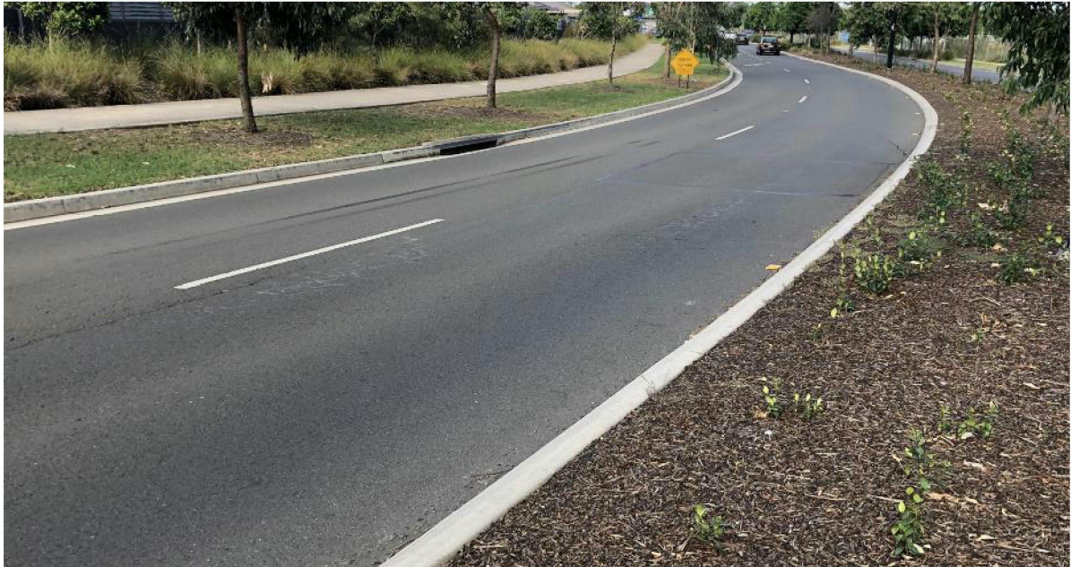
Figure 88: Approx CH250 EB pavement failure (P53)
