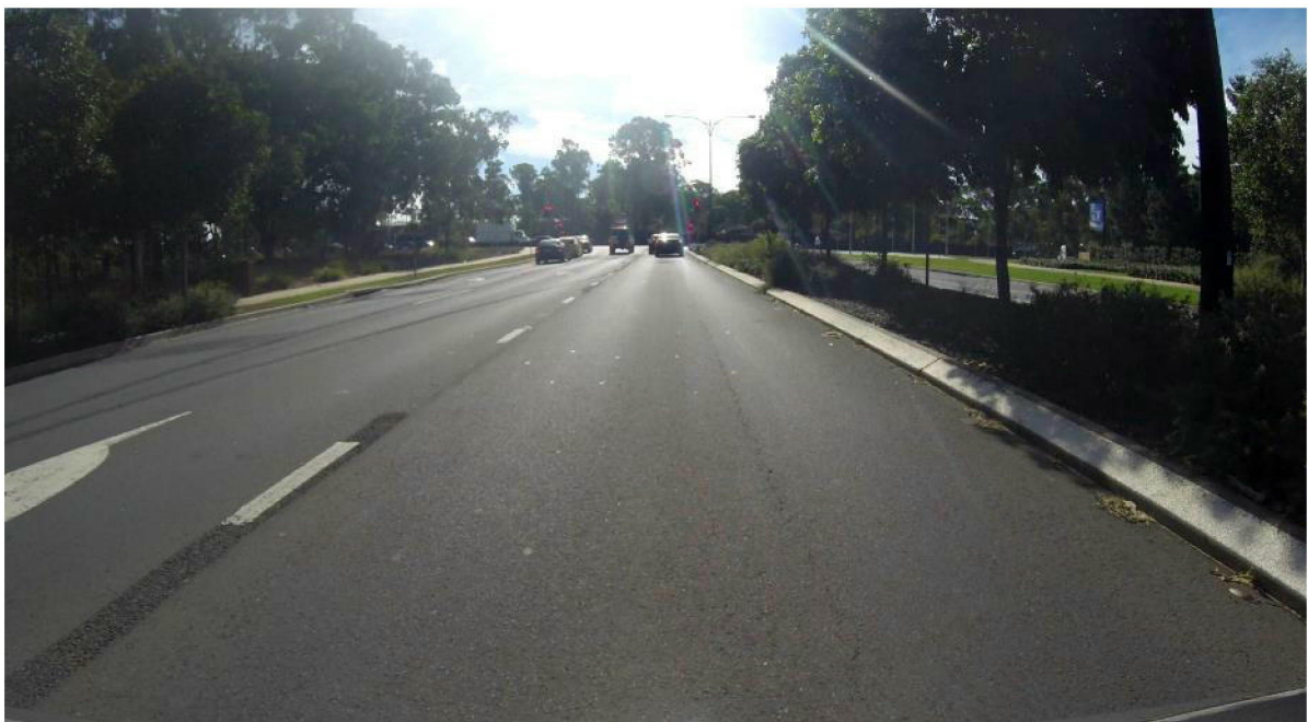
Figure 99: CH440 WB pavement crack/failure
