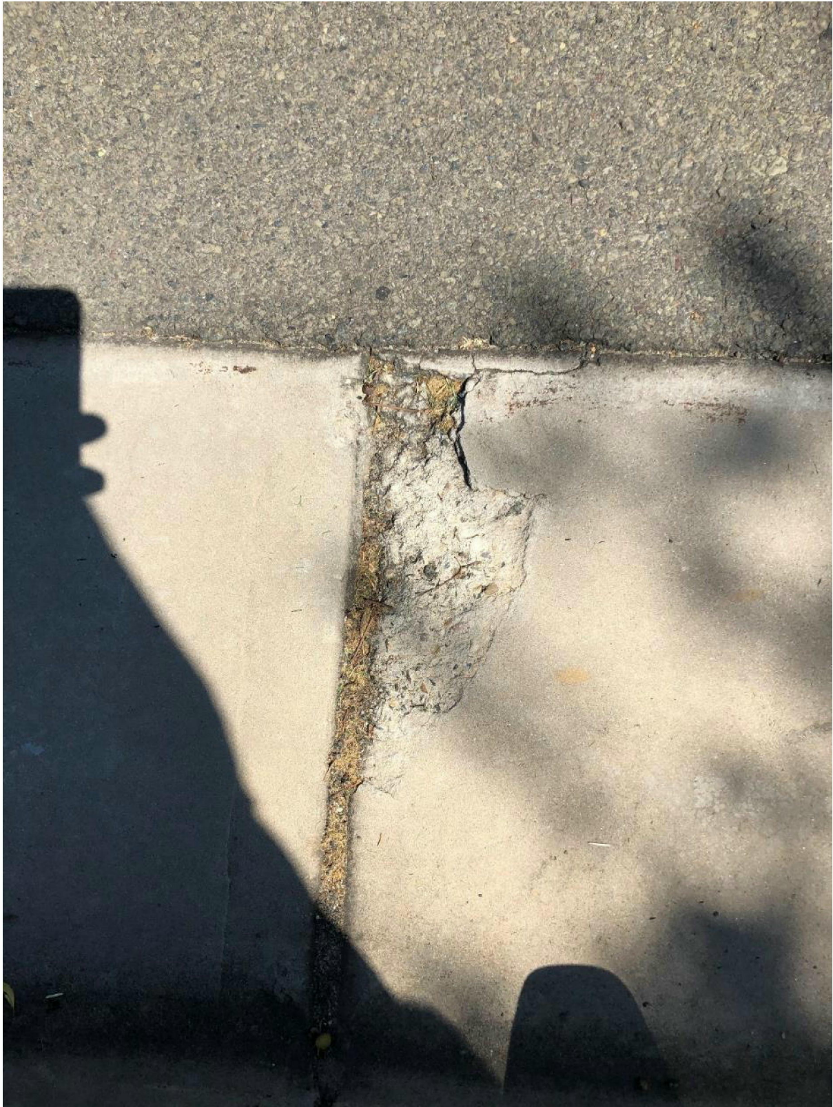
Figure 68: spalling to gutter construction joint interface.
