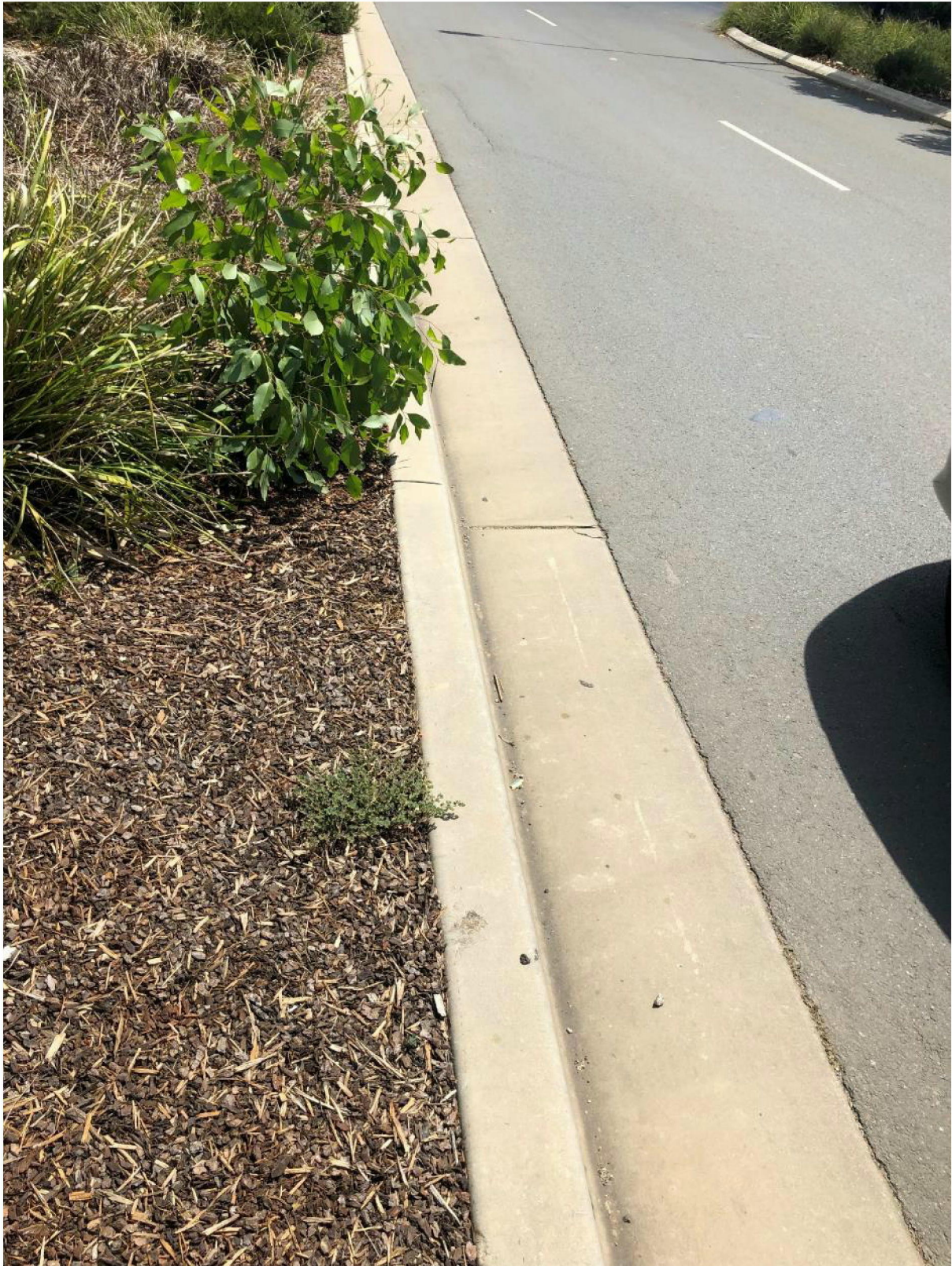
Figure 53: diagonal cracking at construction joint interface.
