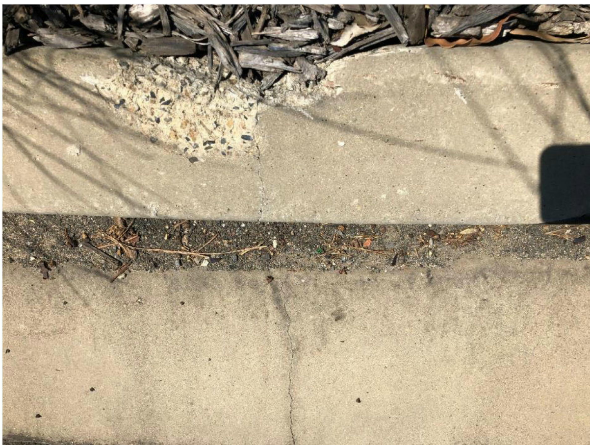
Figure 79: chip to top of kerb.
