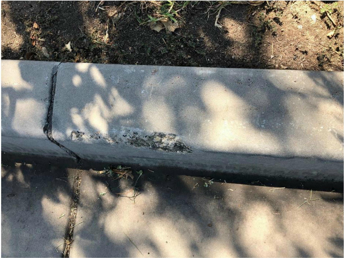
Figure 74: chip to top of gutter.
