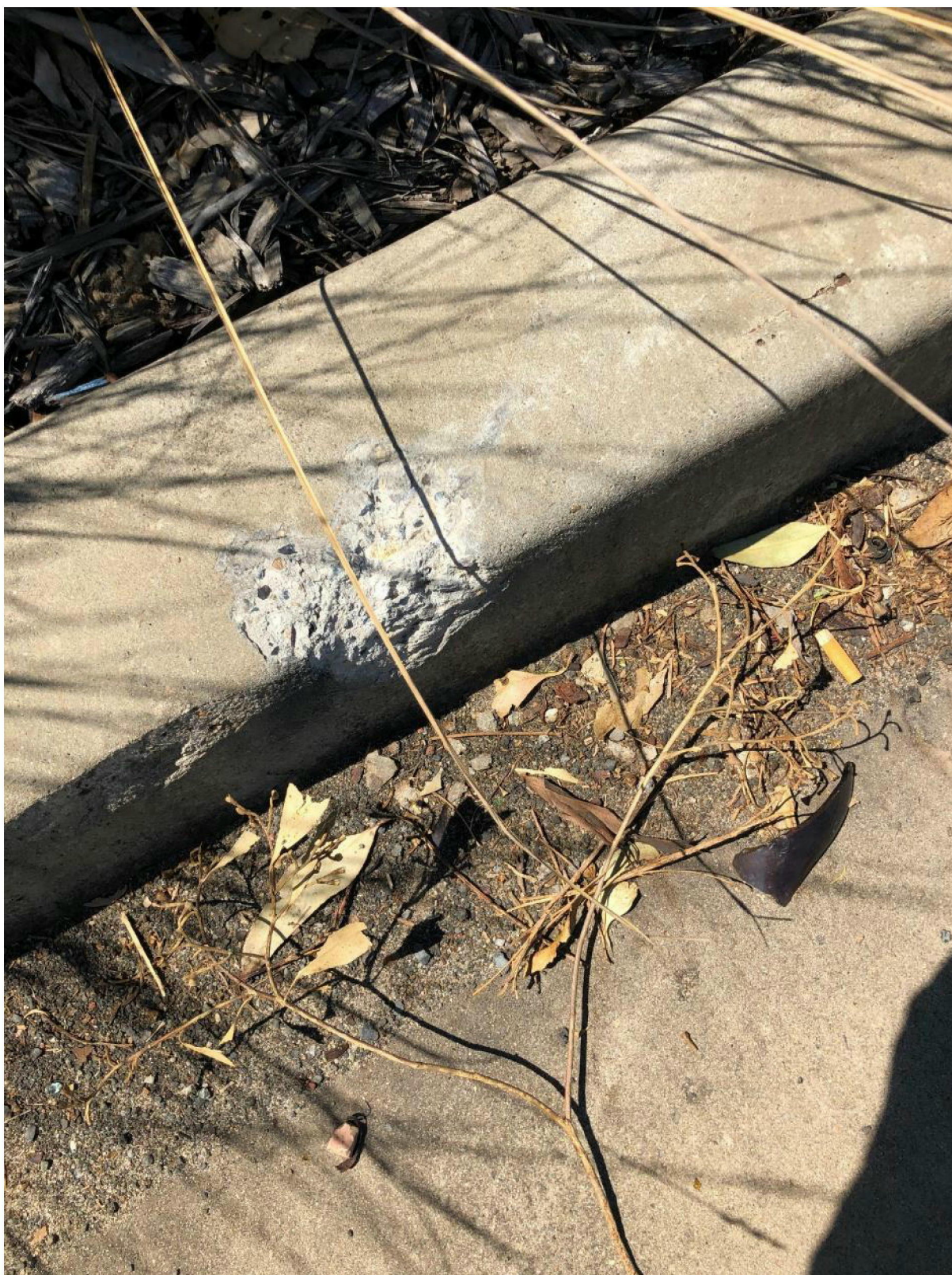
Figure 78: chip to top of kerb.
