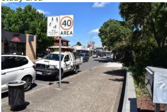
Figure 38. View south-west from the TAFE Building heritage item towards the John Price & Son funeral home within the study area
