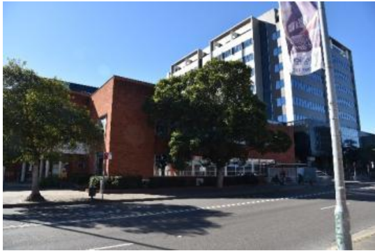
Figure 32. View north-east from Henry Street towards former Council Chambers building (left) and modern development (right)
