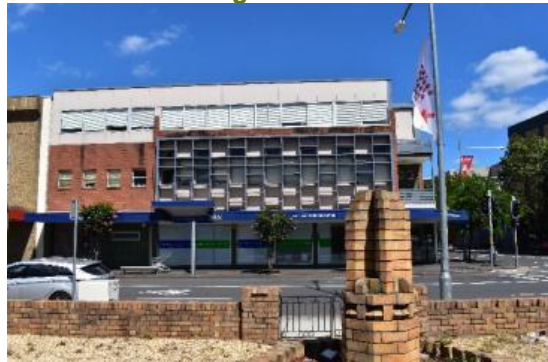
Figure 35. View west from former John Price & Son funeral home towards the former Prospect Electricity building
