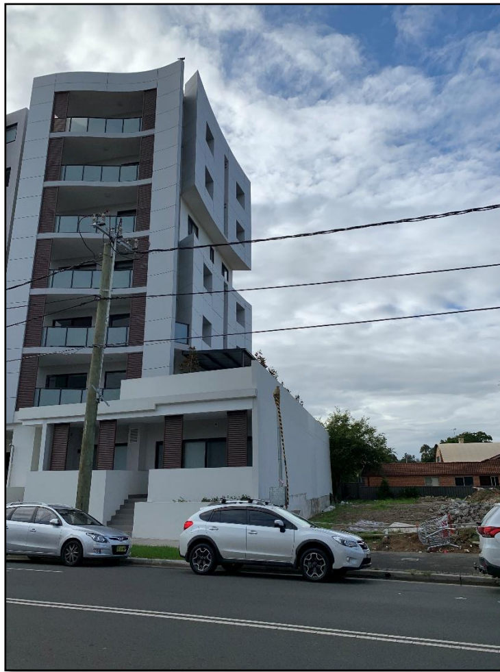
Photograph 3: View of the north-eastern side of the site looking from Station Street and showing the adjoining seven (7) storey residential flat building built to the common boundary at the ground floor level.
