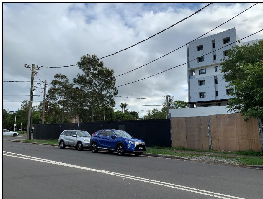
Photograph 2: View of the site looking from Reserve Street.
