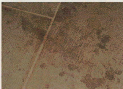
Staining on a historic floor. [©Nicky Ingram]
