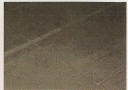
Marks left from the removal of tape attaching druggeting to the floor. [©Nicky Ingram]
