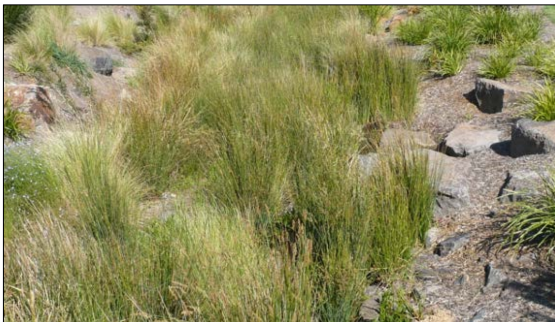
Figure E.1 Typical form of a small vegetated swale Note the Nepean Memorial Park SWMP calls for a 1 in 5 vegetated batter
