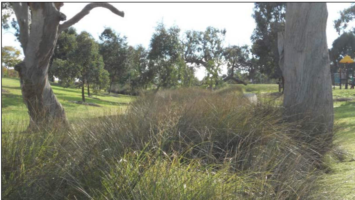
Figure E.2 Typical form of a vegetated swale in Catchment 2
