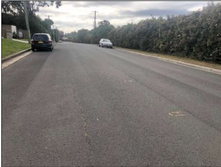
Figure 4a: Park Avenue looking east from the Development Site
