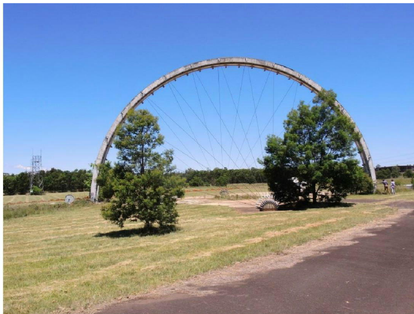
Figure 28 The steel and timber antenna hoop at the former Naval Radar Calibration Range. The figures at right indicate the large scale of this structure. An associated tower is visible in the background at left. Although the hoop is to be demolished, its form could be reproduced in new materials at an appropriate location. (Photo: Chris Betteridge, 18 November 2014)
