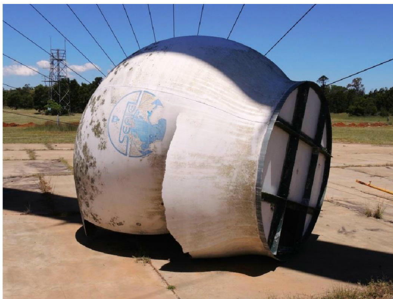
Figure 30 The fibreglass 'Seatel' radome which it is assumed was previously attached to the hoop antenna or one of the other structures on site. (Photo; Chris Betteridge, 18 November 2014)
