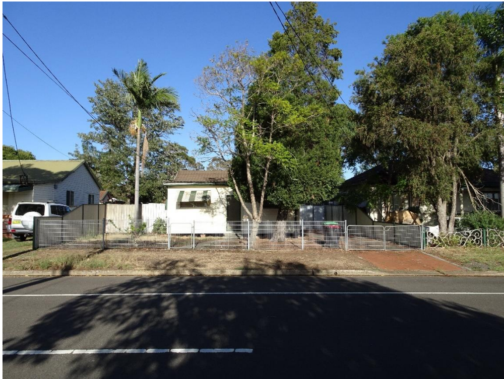
Figure 3b: Photograph of 11 Sydney Street from Sydney Street
