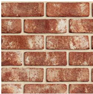
05 recycled brick external walls & subfloor
