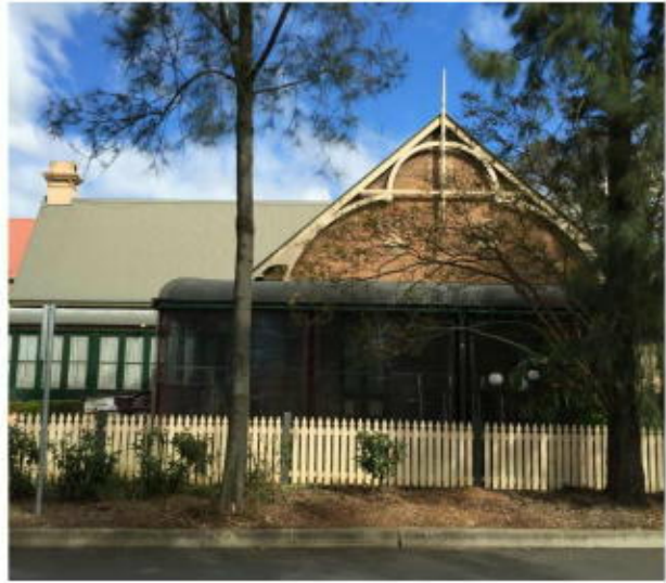
PICTURE 2 – EASTERN FAÇADE OF 146 STATION STREET
