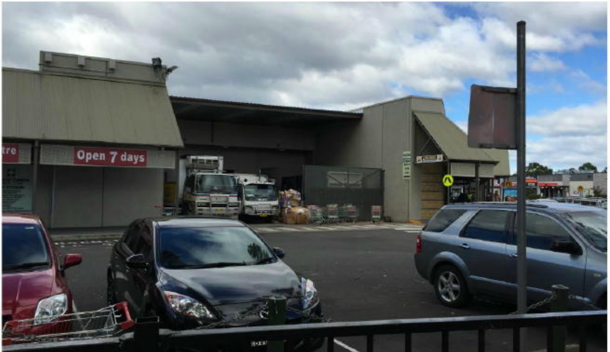
FIGURE 4 – VIEW OF THE LOADING DOCK AND CAR PARK
