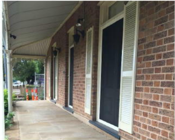
PICTURE 4 – VERANDAH AT 148 STATION STREET
