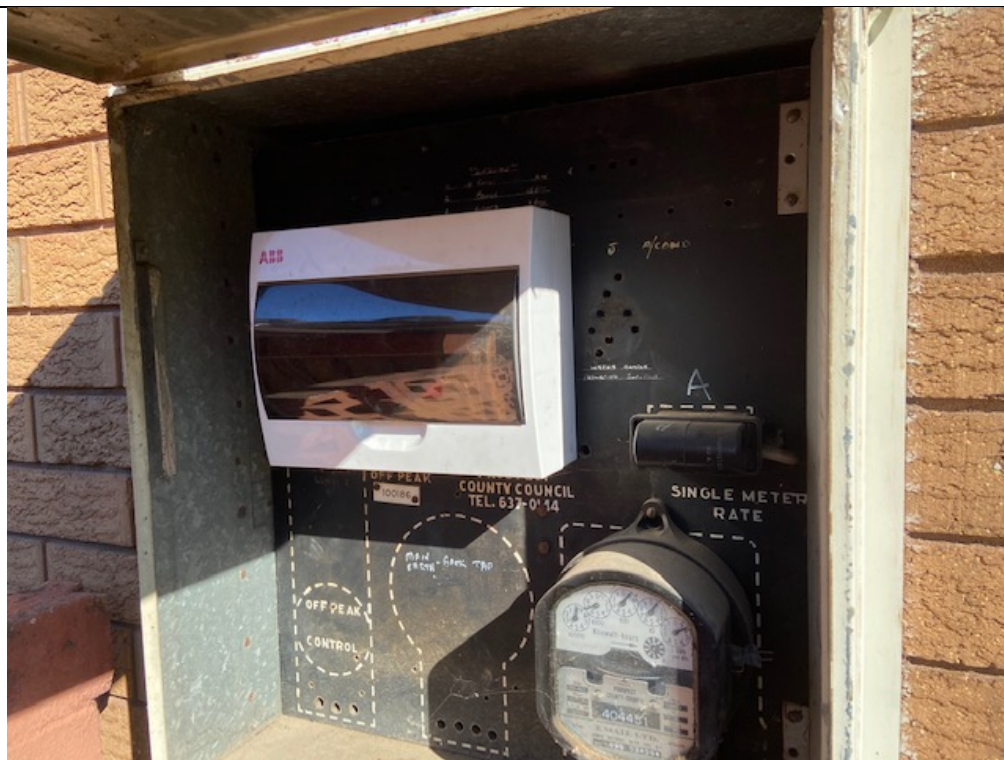
Photo 14 – Lot 51 – 22 Rodley Av., Penrith; Residential Dwelling; Hazardous Building Materials Deemed to Exist within Building Fabric (e.g. Asbestos-Based Phenolic Backing Board to Electrical Meter Box)
