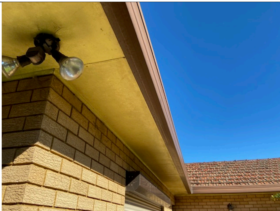
Photo 5 – Lot 52 – 24 Rodley Av., Penrith; Residential Dwelling; Hazardous Building Materials Deemed to Exist within Building Fabric (e.g. Asbestos Cement Eave Sheeting)
