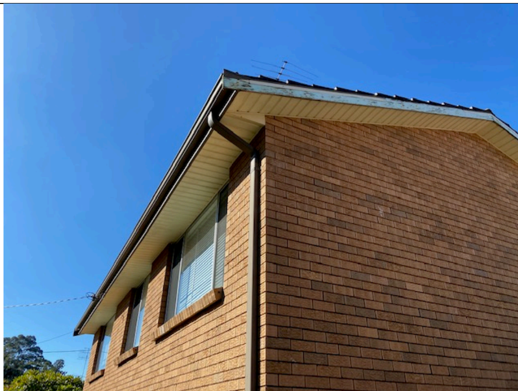
Photo 13 – Lot 51 – 22 Rodley Av., Penrith; Residential Dwelling; Hazardous Building Materials Deemed to Exist within Building Fabric (e.g. Asbestos Cement Eave Sheeting [above vinyl overlay] & Roof Tile Support Panels)
