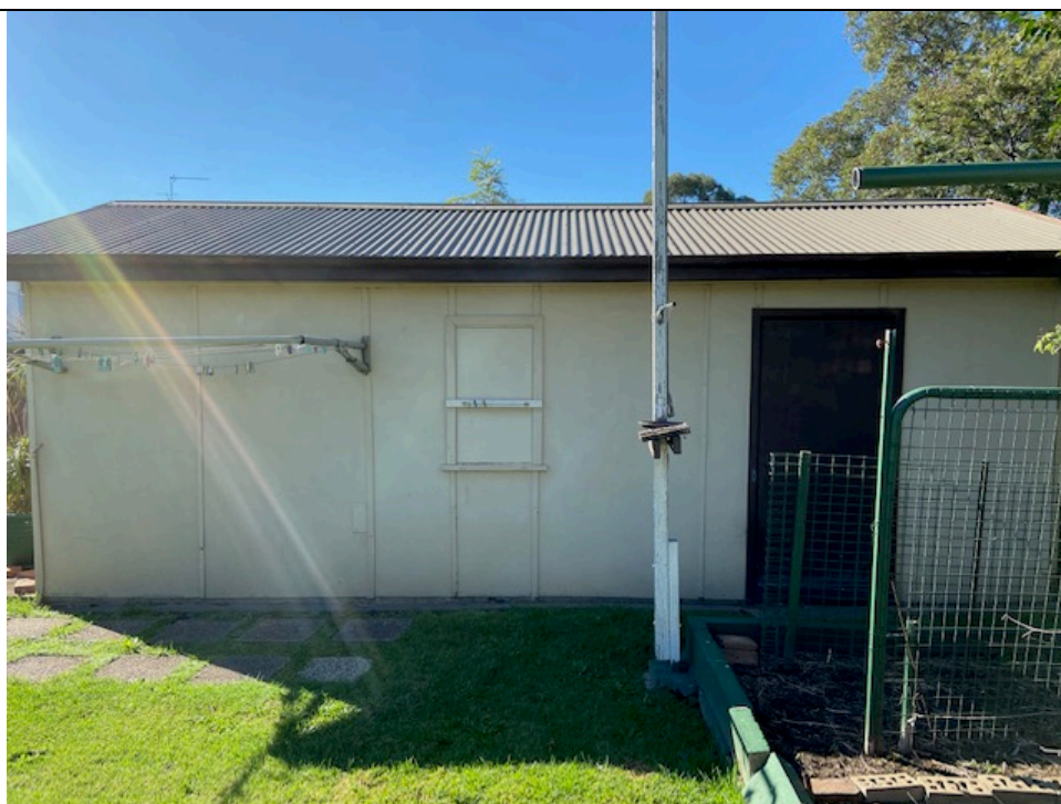
Photo 6 – Lot 52 – 24 Rodley Av., Penrith; Detached Garage to Rear Yard; Hazardous Building Materials Deemed to Exist within Building Fabric (e.g. Asbestos Cement Exterior Cladding)
