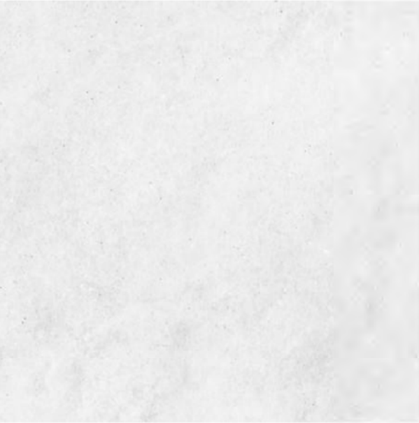
WHITE PAINTED PRECAST
