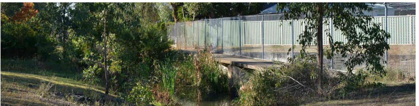
View 4 - Looking south-east at existing box culvert and Werrington Downs residential boundary. Stitched using 50mm focal length.
