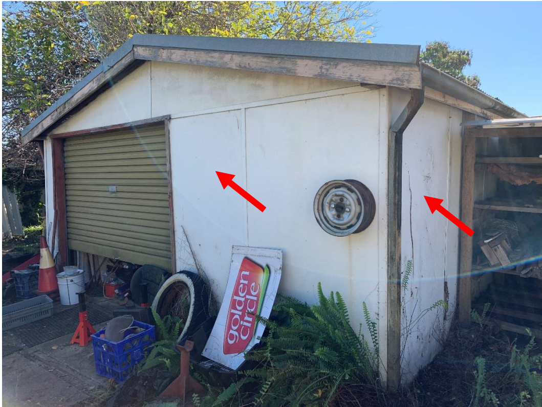
Photo 23: Showing exterior walls of garage at 42 Mamre Road, St Marys NSW, contains ACM.
