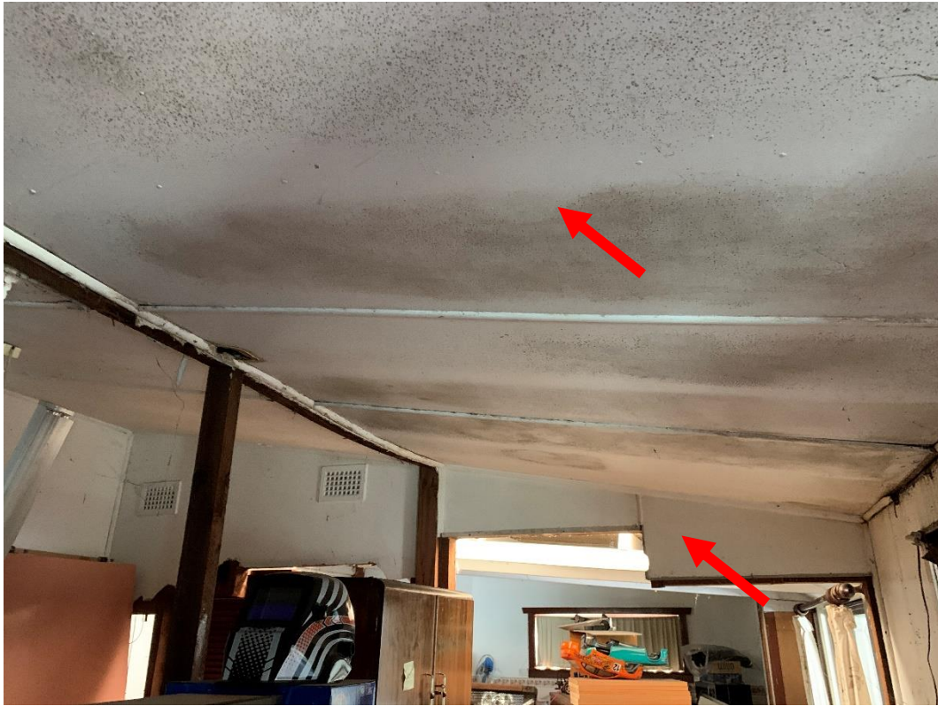
Photo 15: Showing interior sunroom walls and ceiling at 42 Mamre Road, St Marys NSW, contains ACM.
