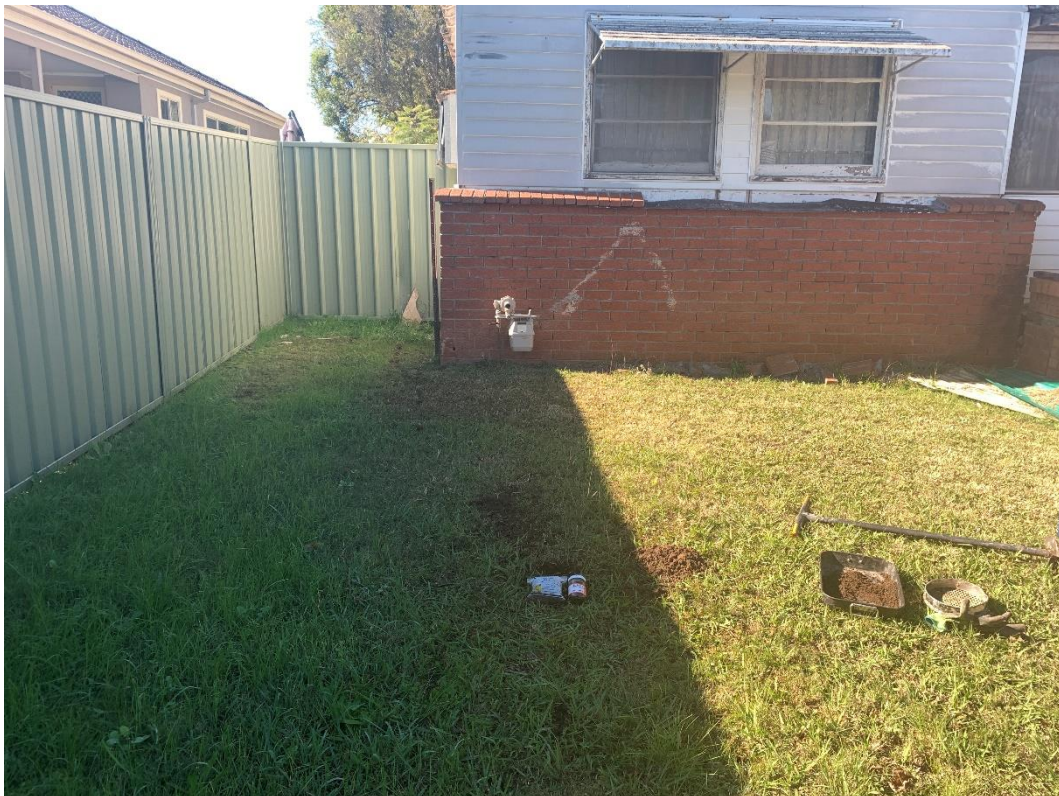
Photo 4: Showing borehole BH2 sampling location, 42 Mamre Road, St Marys, looking east.
