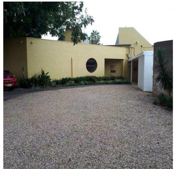
Carpark North view – Gallery carpark entrance
