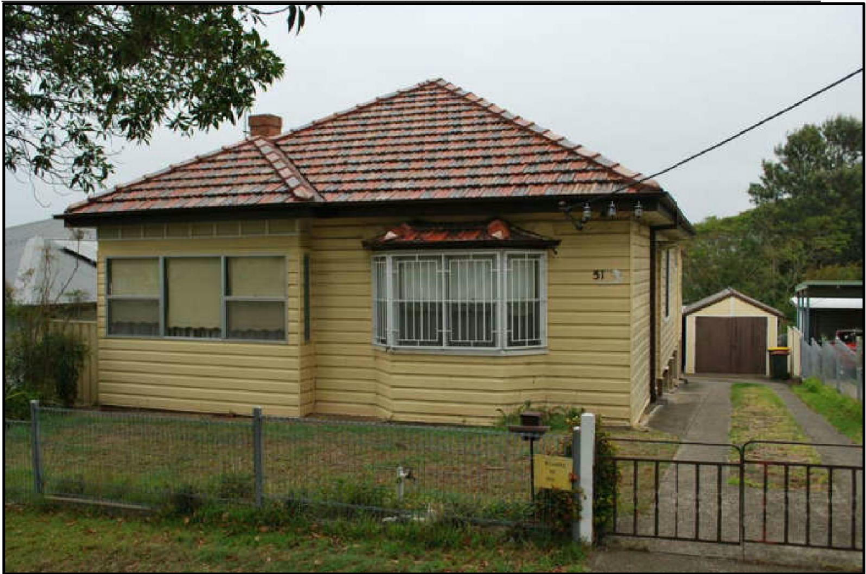
Figure 4 Building to be relocated at current location
