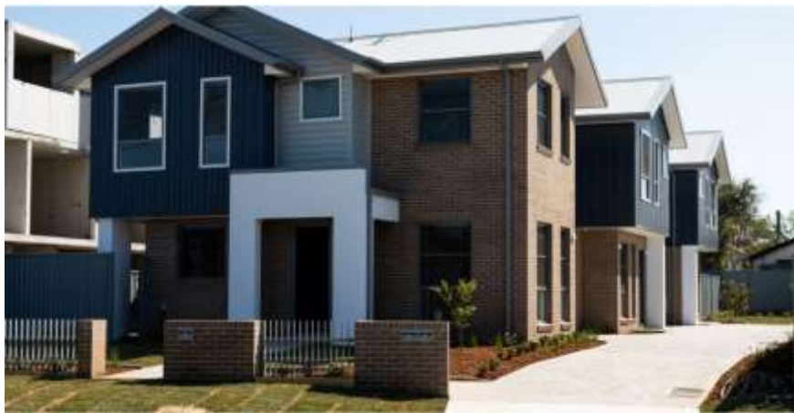
The image above shows the recently constructed two-storey townhouses at 44 Park Avenue approved under DA18/0292.
