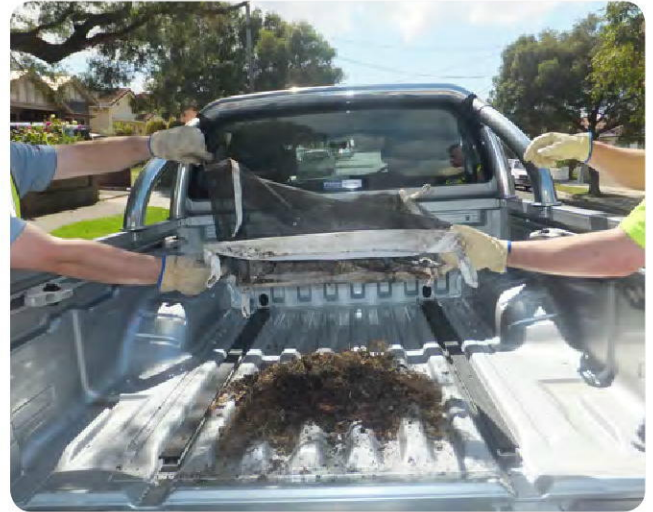
Photo 26 A clean used filter bag
