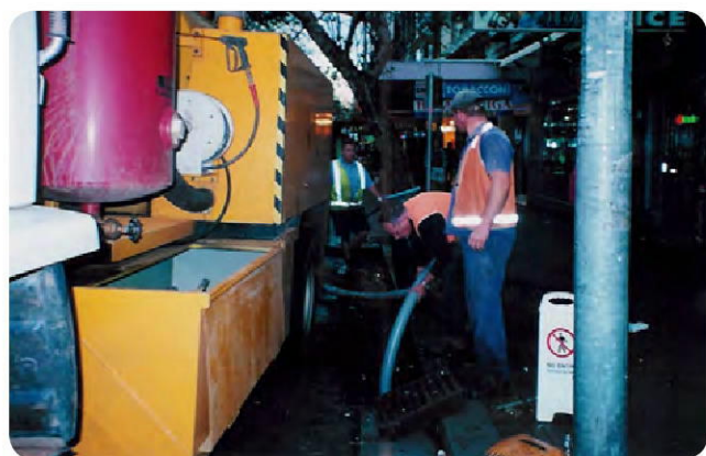
Photo 11 Cleaning an EnviroPod using the inductor method
