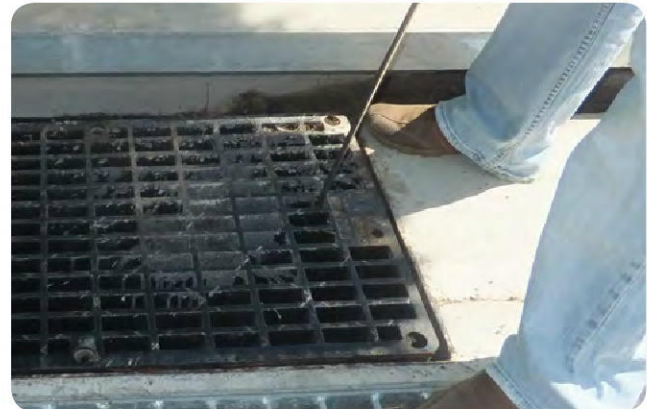
Photo 6 Insert hook near edge of grate
