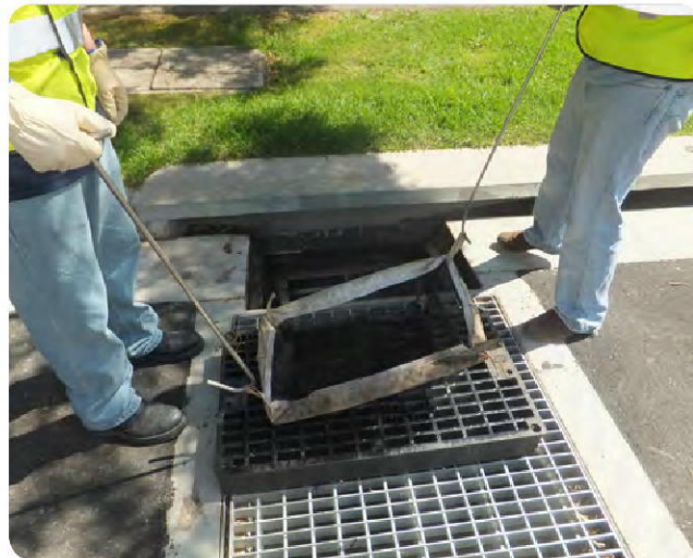
Photo 19 Reinstall filter bag
