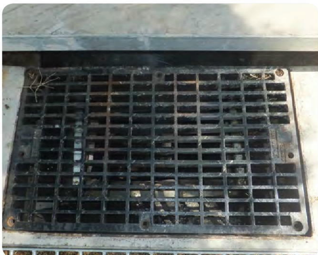
Photo 22 Installed filter bag and sealed pit
