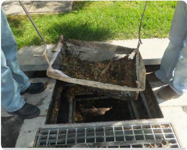
Photo 14 Lift the bag from the stormwater pit
