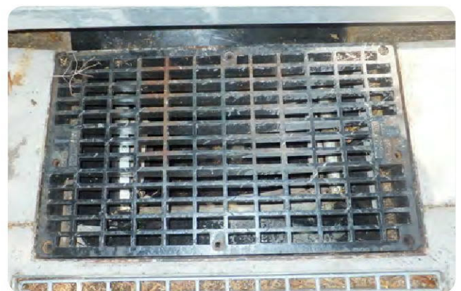
Photo 10 Reinstated non hinged grate
