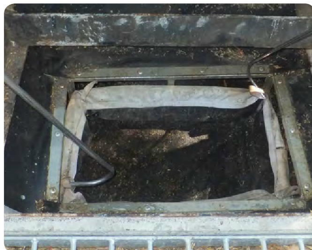
Photo 21 Correctly installed filter bag
