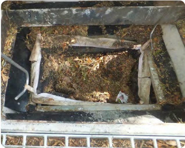
Photo 12 Place the lifting hooks through the bag loops
