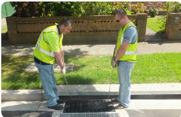
Photo 7 Position each lifter either side of the grate
