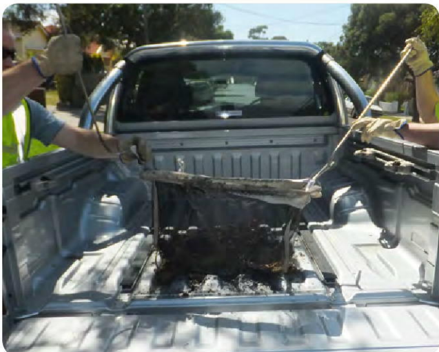
Photo 16 Grab the bottom lifting loops
