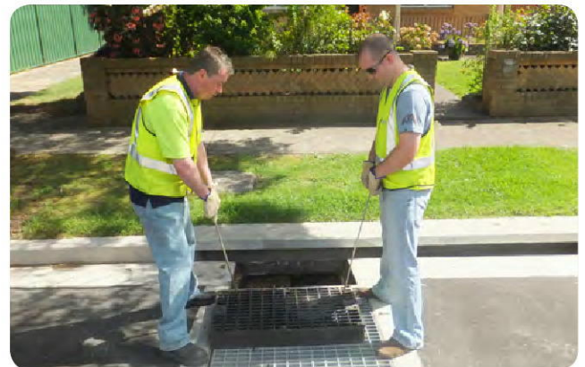
Photo 8 Lift grate and move grate to one side
