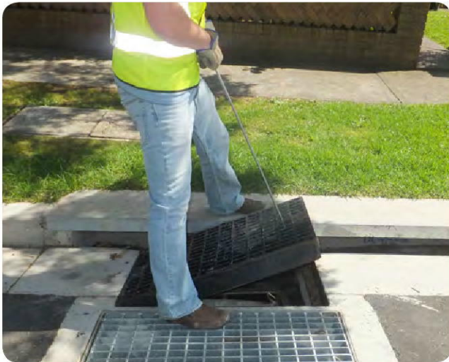
Photo 3 Lifting the grate
