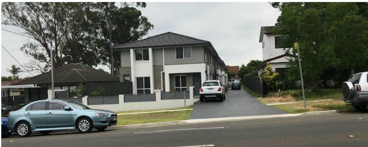
Figure 9. View of 153 Jamison Road (Viewing North)
