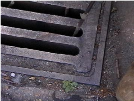
Plate 6 Insert hook near edge of grate
