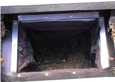
Plate 22 Correctly installed filter bag
