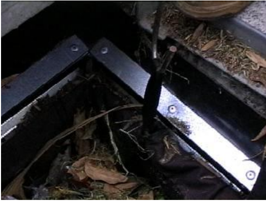
Plate 12 Place the lifting hooks through the bag loops
