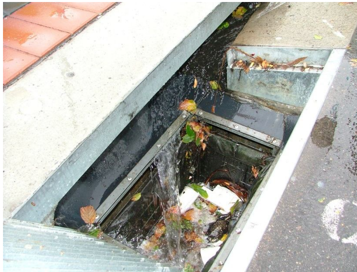
Enviropod filter in service.
