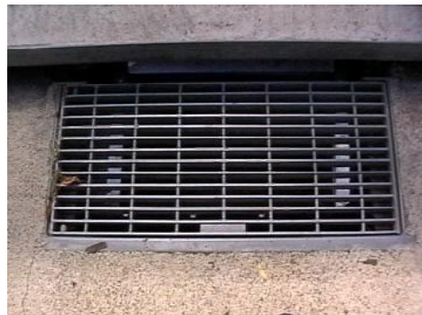
Plate 23 Installed filter bag and sealed pit
