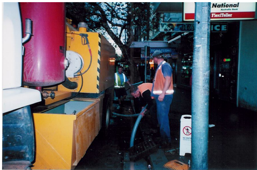
Plate 11 Cleaning an Enviropod using the inductor method
