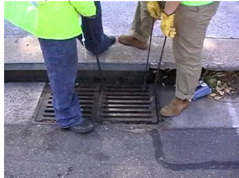
Plate 7 Position each lifter either side of the grate
