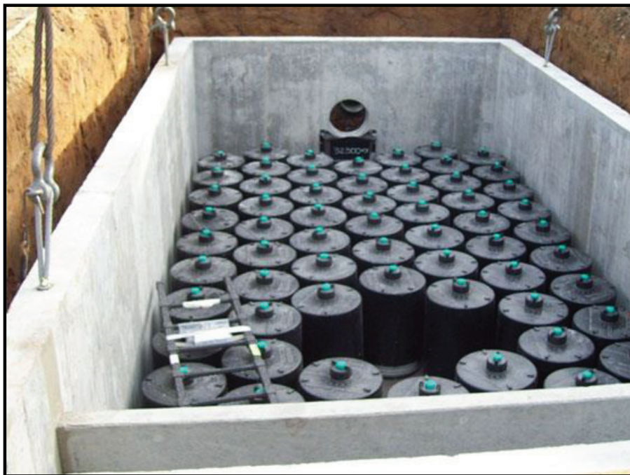
Plate 5.1 - Typical Cartridges Filter System (During Construction)
