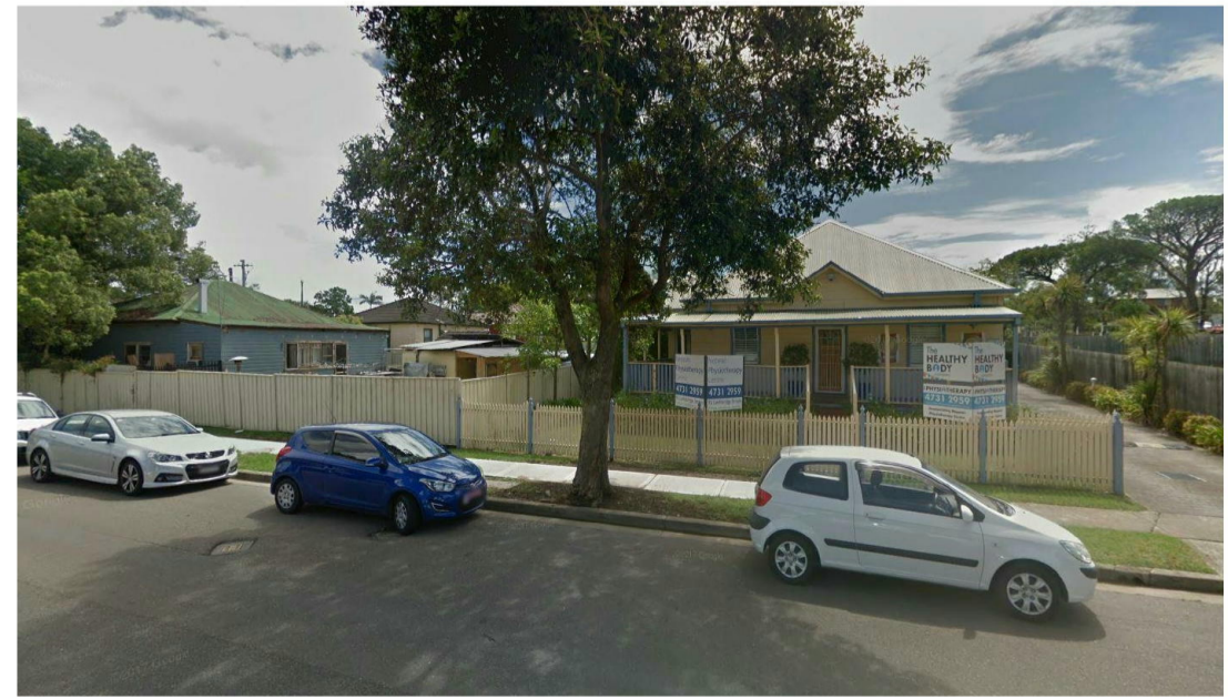
95 LETHBRIDGE ST - EXISTING SINGLE STORY DWELLING
