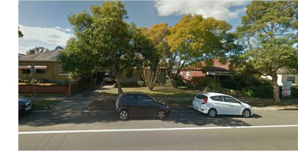
32 EVAN ST - EXISTING SINGLE DWELLING TO BE DEMOLISHED
