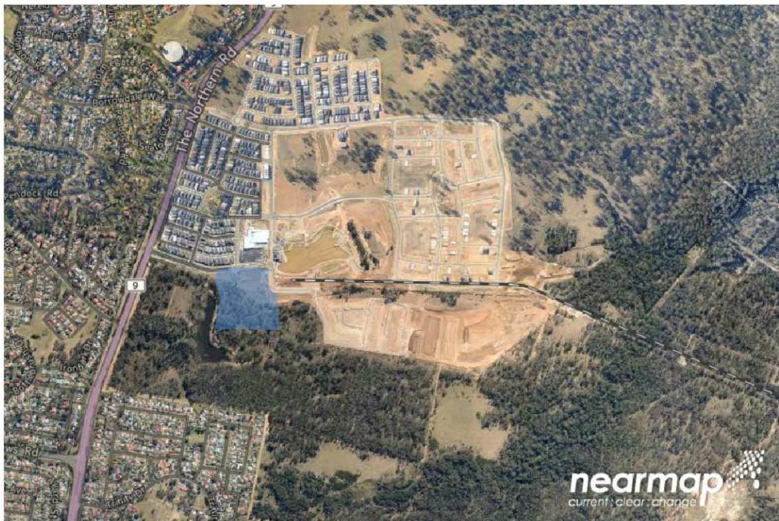
Figure 1.1: Subject Site and its Environs
