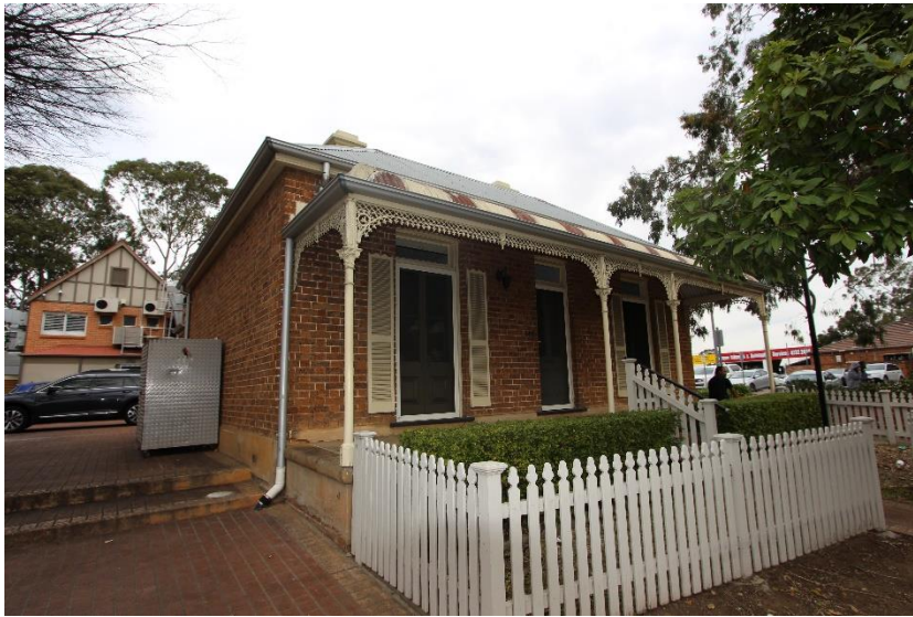
Figure 5: View of 146 Station Street taken from across the road
