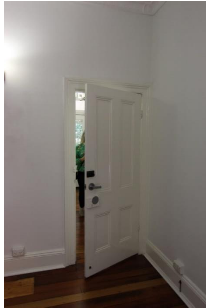
Figure 24: Four paneled internal door
