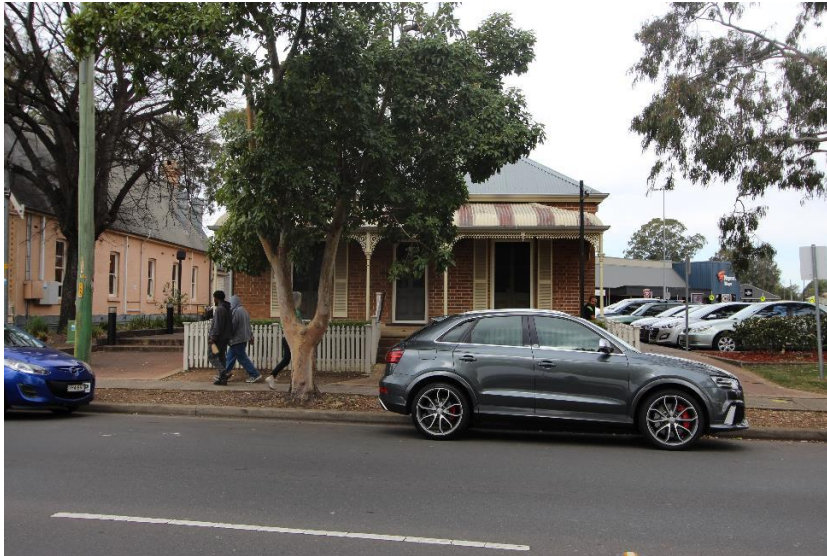
Figure 9: View of 148 Station Street taken from across the road
