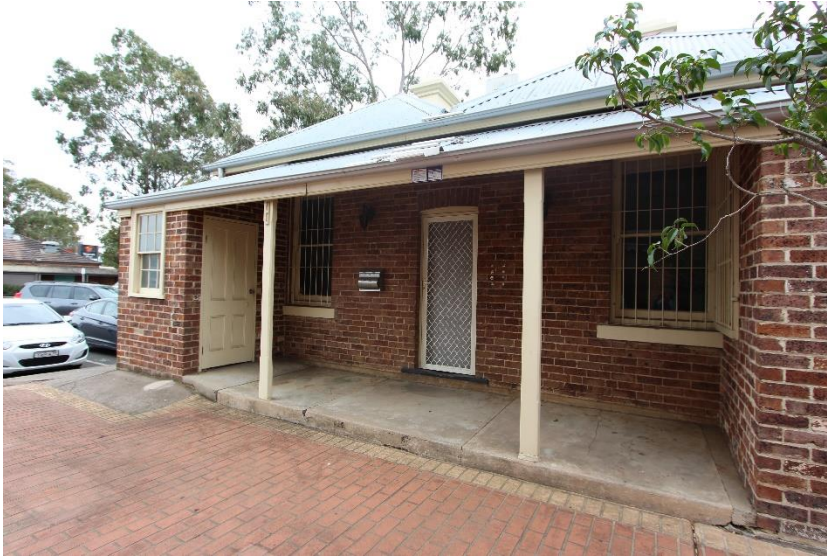
Figure 17: The rear facade
