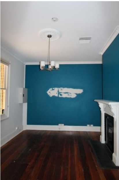
Figure 25: Rear western side room
