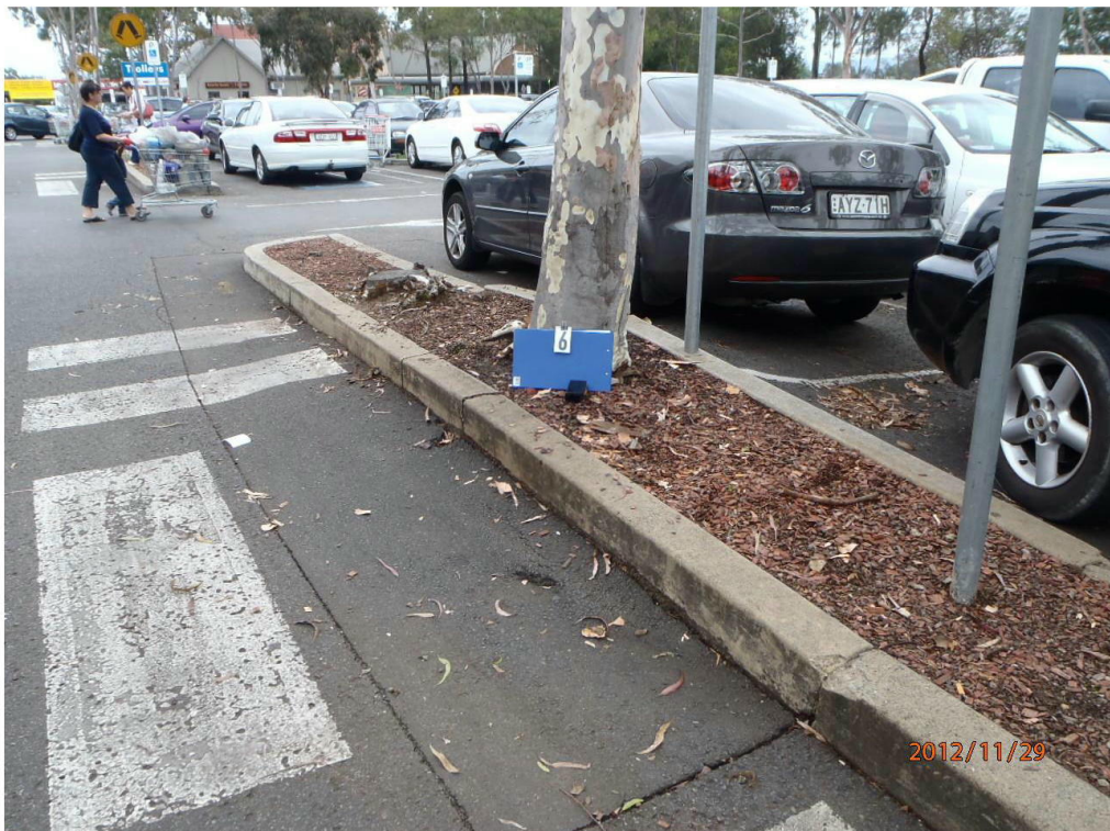
Plate 4: Another example of repairs within the SRZ distance on Tree 6. P. Vezgoff.
