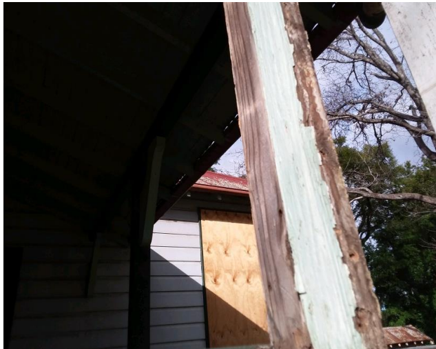
Notes: Close-up visual inspection to the removal area following removal
