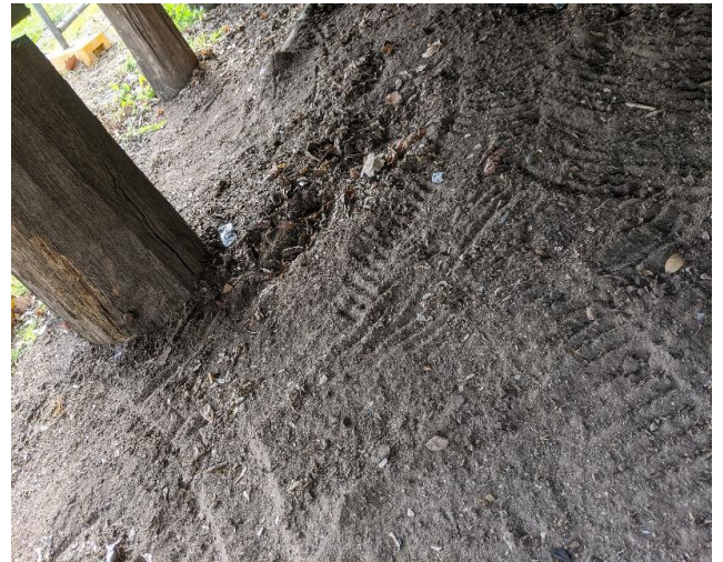
Notes: Overview of remediation area (subfloor) following remediation
