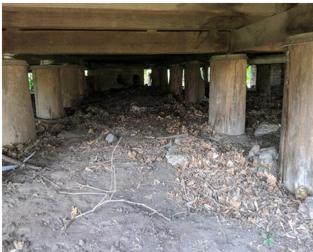
Notes: Overview of remediation area (subfloor) following remediation
