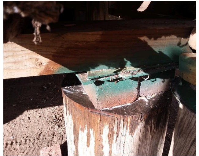
Notes: Visual inspection to the packing material following encapsulation
