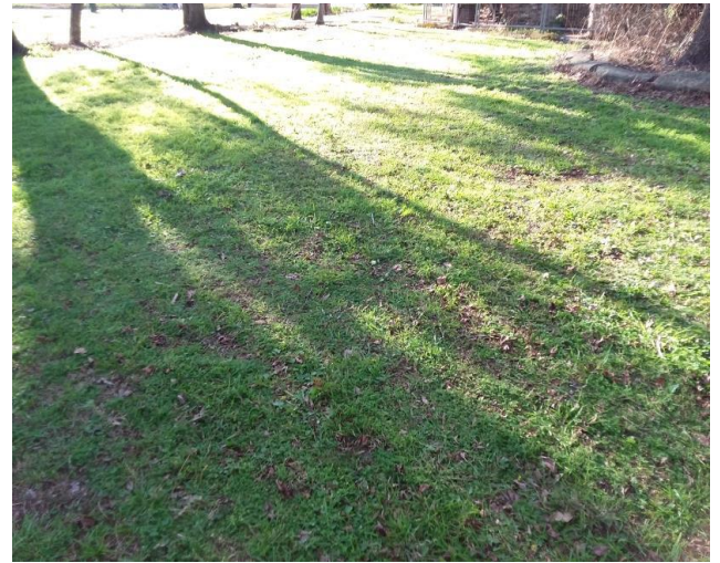
Notes: Visual inspection to the top surface of vicinity of remediation area
