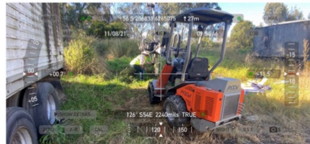
Photo 11: Drilling at BH10 at Stockpile 2
