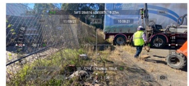
Photo 12: Drilling at BH4
