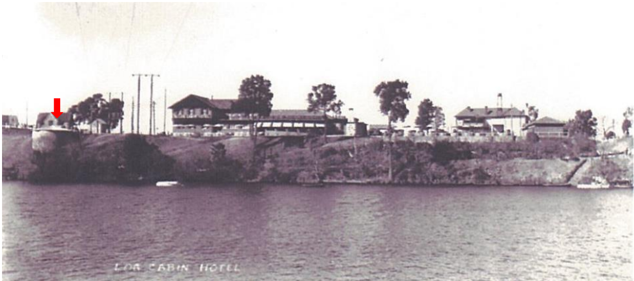
Figure 48 – Photograph, c1940, of the subject site from the western side of the river. Including a clear image of the remnant pump house with what appears to be a flat roof (indicated).
