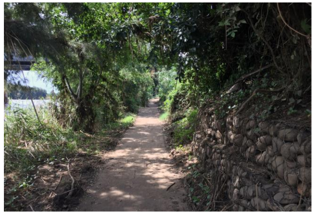
Figure 34 – View north-east along the public walkway along the riverbank, located west of Lot 21.
