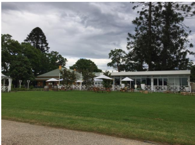
Figure 41 – View west towards “Emu Hall” including contemporary addition.
