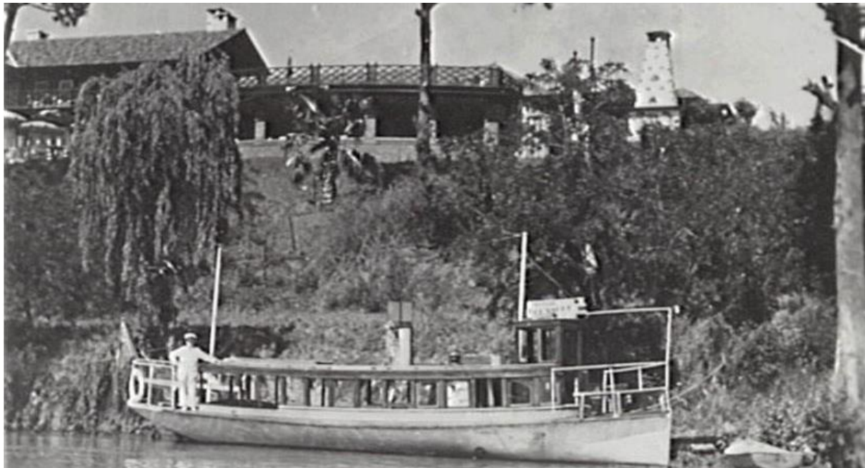
Figure 65 – 1940s photograph showing the Ferry Crossing, with the Log Cabin visible in the background.
