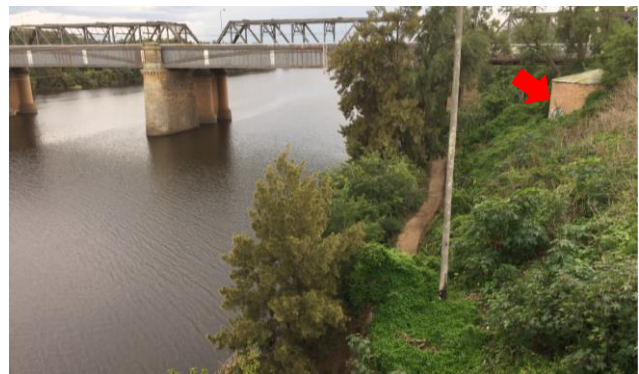
Figure 38 – View north-east from the Yandhai bridge down to the approximate location of heritage item no: 870. The remnant Pump House is seen on the right (indicated) and both Victoria Bridge and Underbridge in the background.
