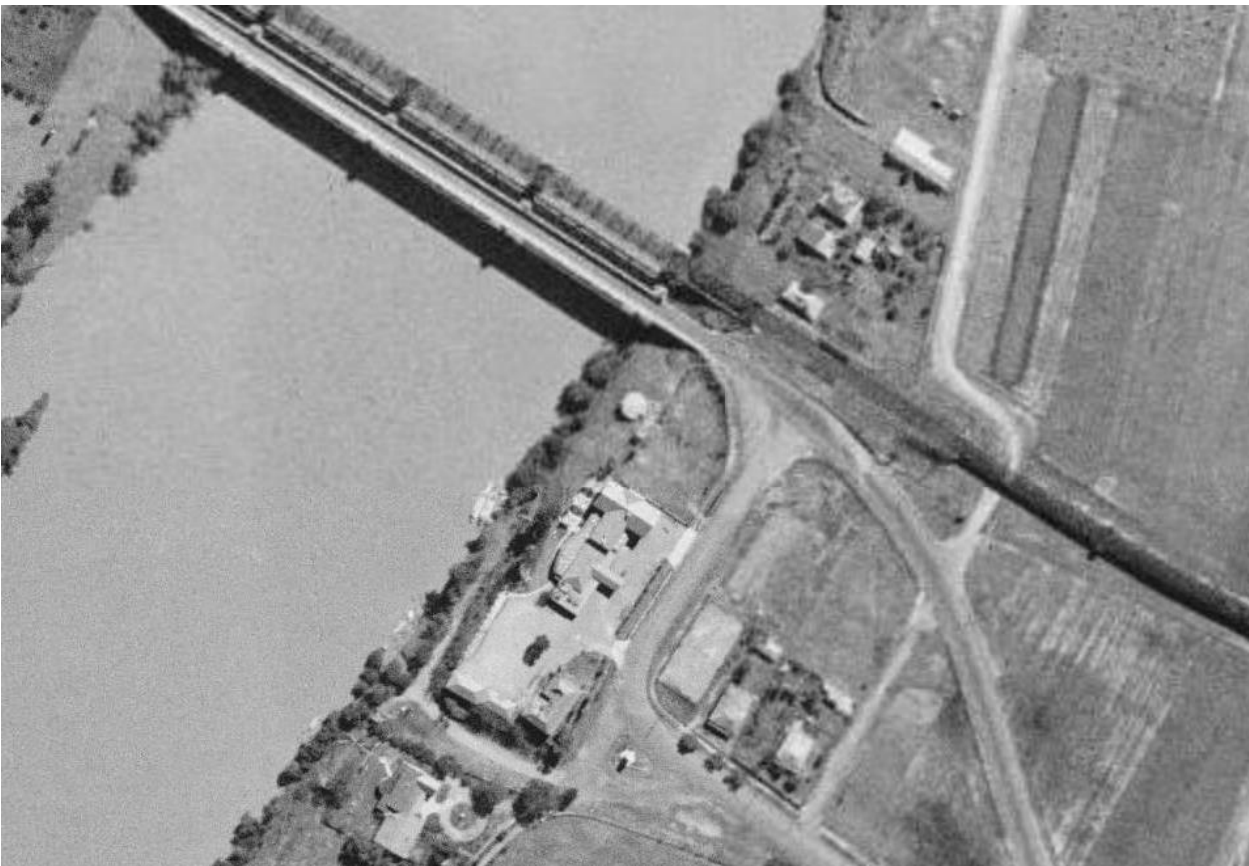
Figure 58 – 1943 aerial showing the Log Cabin and water tank/pump (present on the subject site). This was prior to the construction of the water treatment plant.
