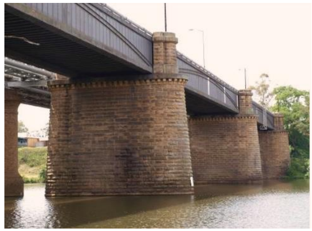
Figure 30 – Sandstone piers at the eastern end of Victoria Bridge.
