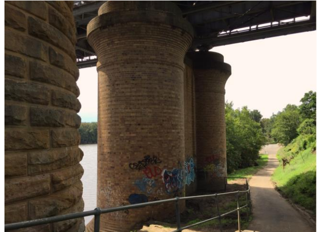
Figure 28 – Brick piers beneath the railway line.
