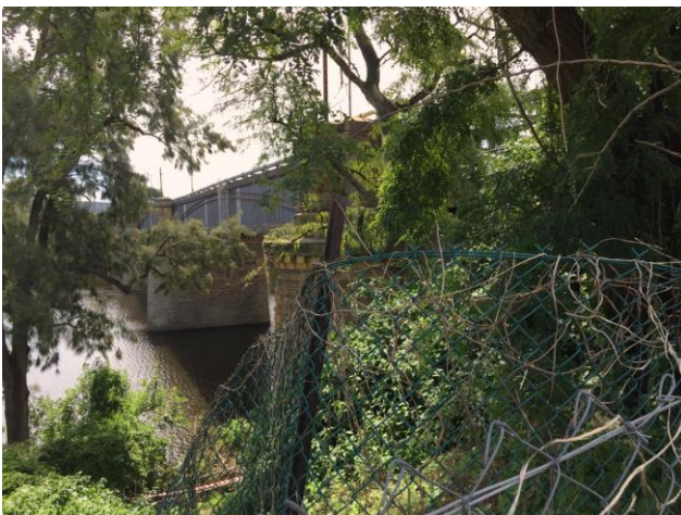
Figure 29 – View of Victoria Bridge from the northern corner of the Lot 21
