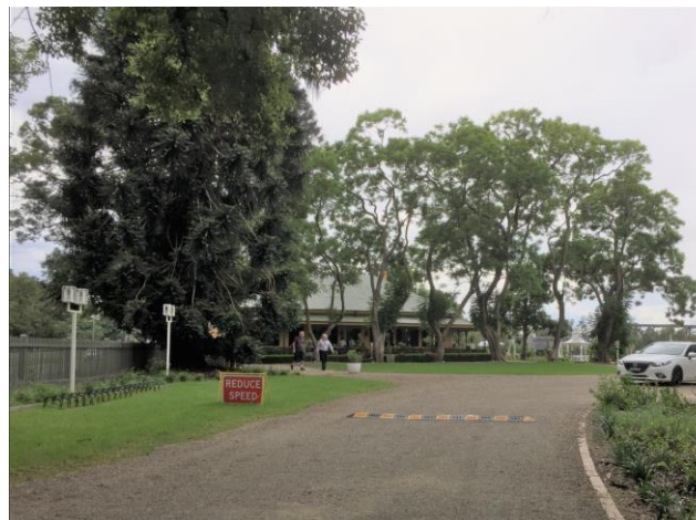
Figure 42 – View north-east from the vehicular entrance to “Emu Hall”.
