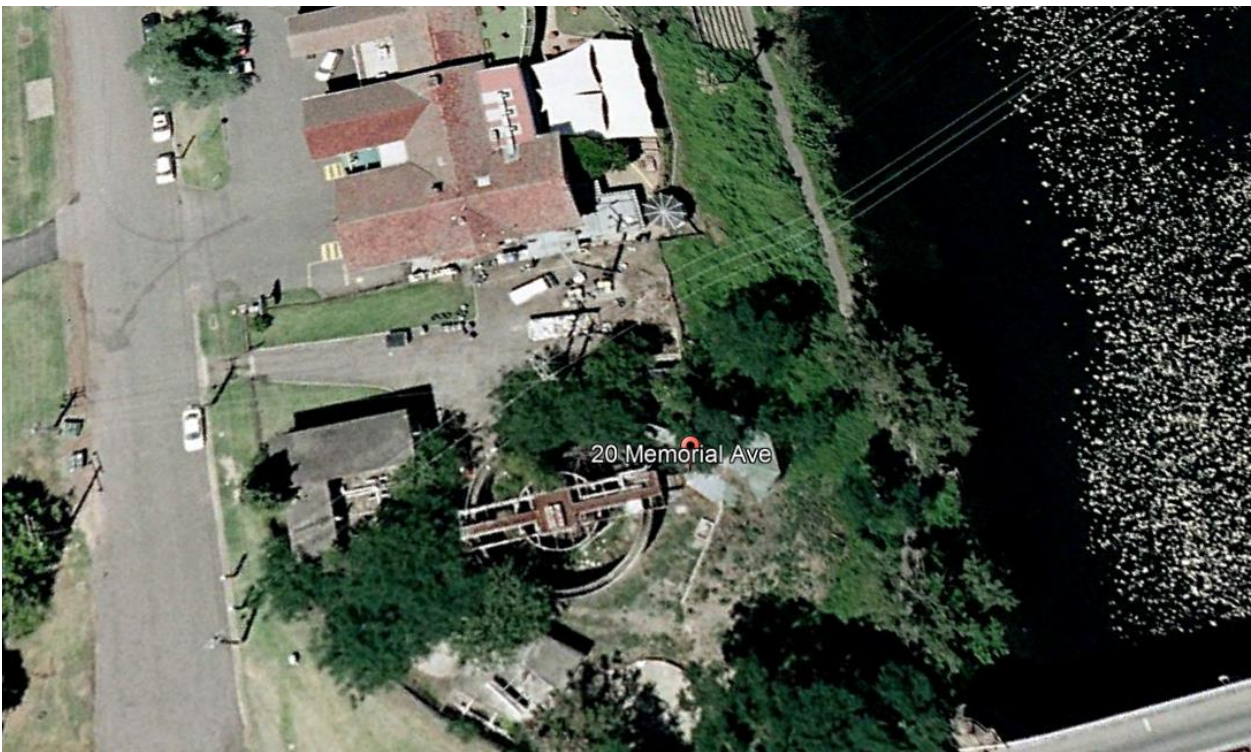
Figure 54 – 2009 aerial view of the water treatment plant – showing the use/location of the remaining tank.
