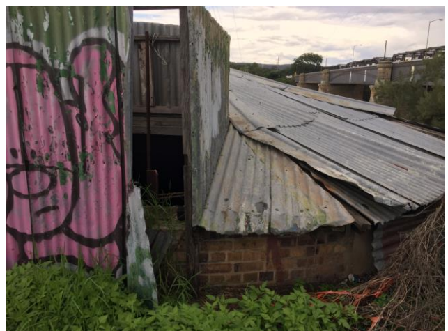
Figure 20 – Later addition roof of the remnant Pump House.
