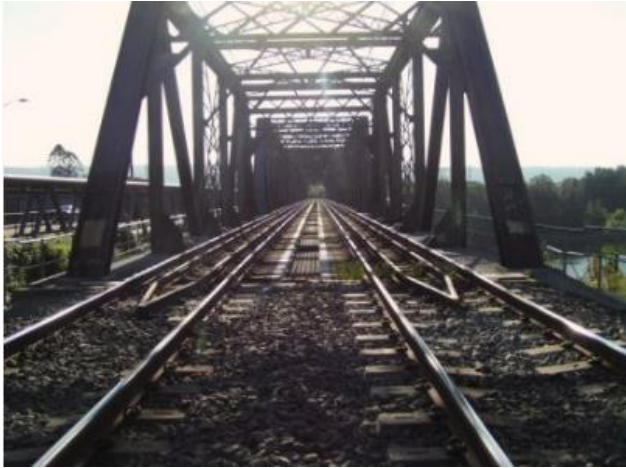
Figure 27 – View west along the Emu Plains Underbridge.
