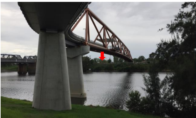
Figure 37 – View from the western side of the Nepean River. Approximate location of heritage item no: 147. The location of the subject site is indicated in red.
