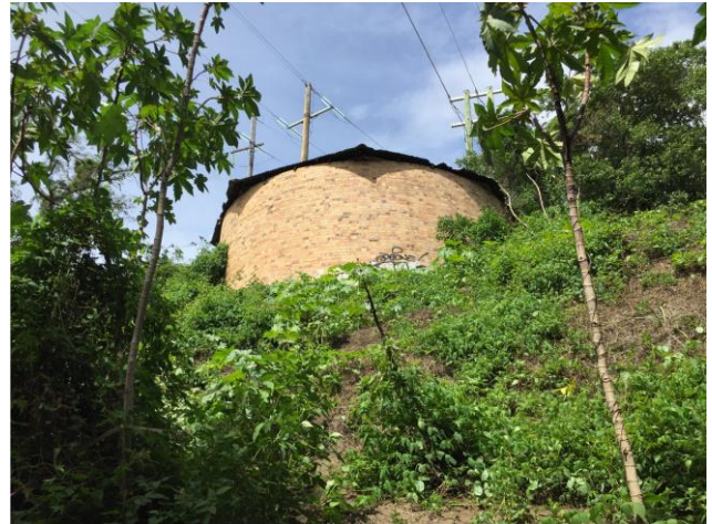
Figure 18 – View of the former Pump House looking east from the riverbank.
