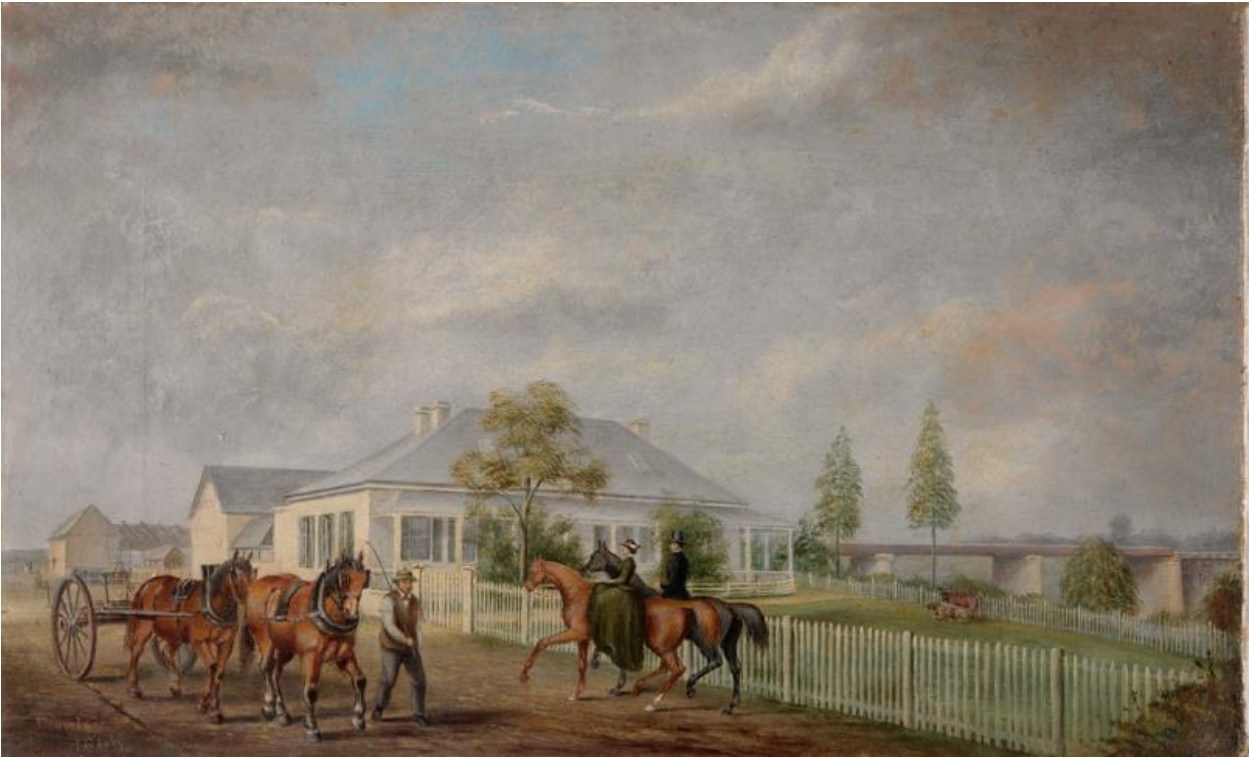
Figure 68 – Painting of Emu Hall by Joseph Fowles - 1866. Note this is prior to the construction of the Underbridge. Victoria Bridge is visible at right.
