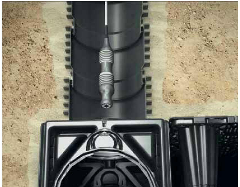
Inspection cameras are introduced into the system through the access shaft.
