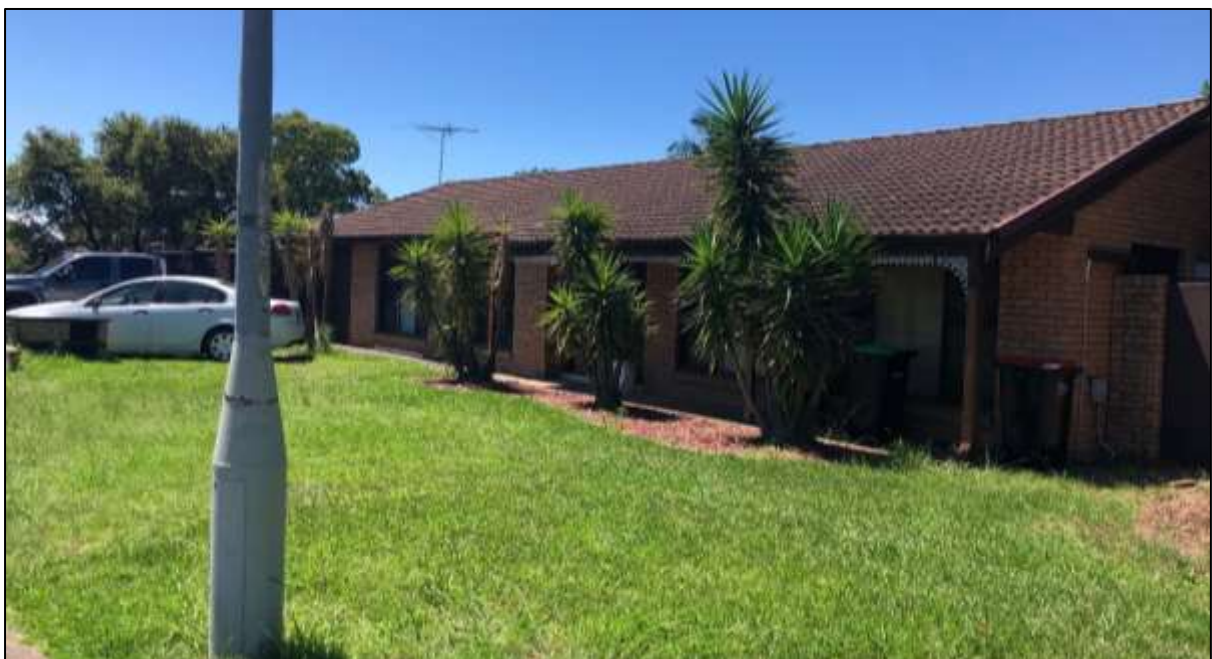
Figure 1: 194 Bennett Road facing North. Source: L. Gibson January 2021.
