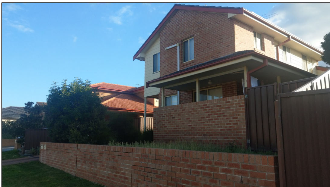
Figure 19: Townhouse development at 28 Edward Street
