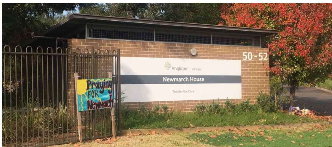
Figure 1.5: Entrance to Newmarch House from Manning Street
