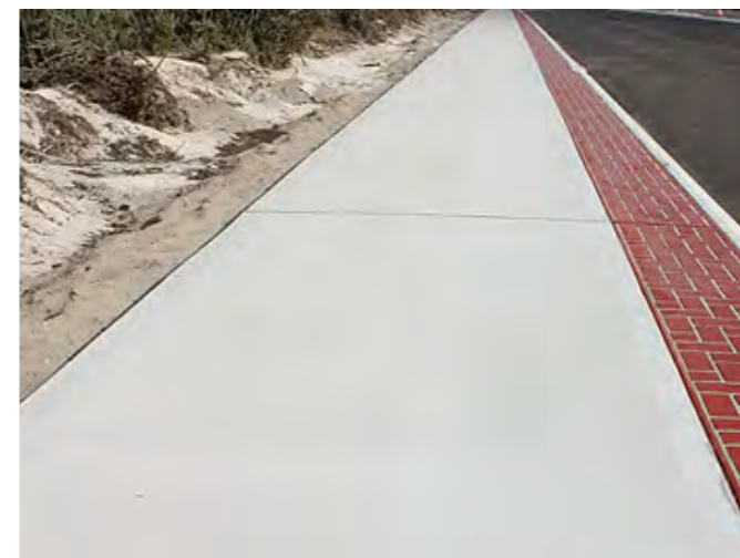
Broom finished concrete shared user path
