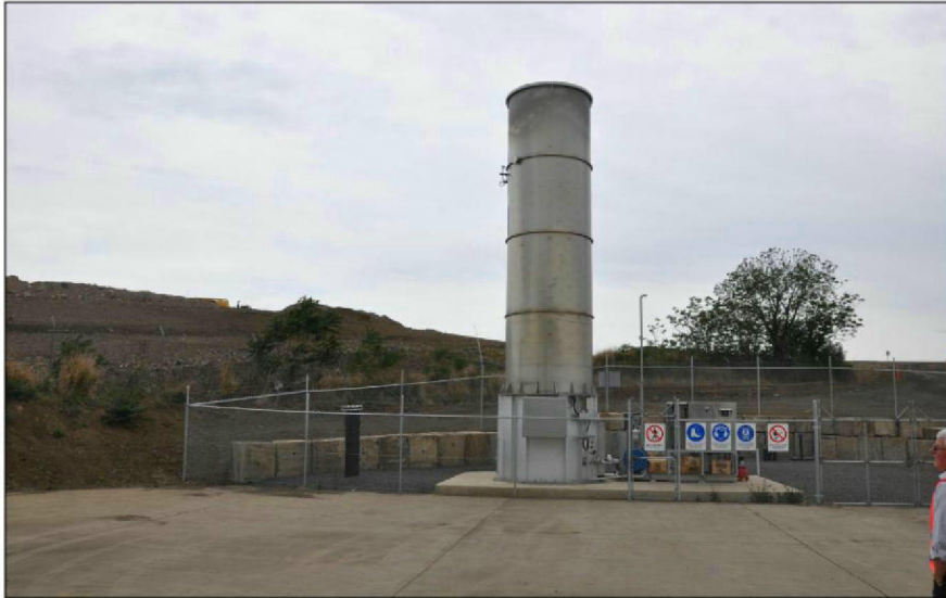
Plate 1.1: Existing Erskine Park Waste Management Facility flare and exhaust stack (Ref: E863B/001)
