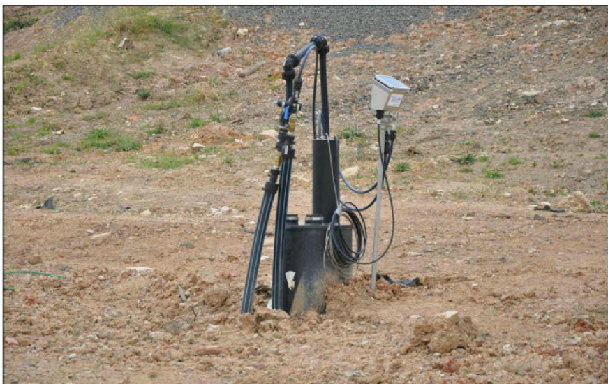
Plate 1.3: Existing landfill gas collection bore (Ref: E863B/009)
