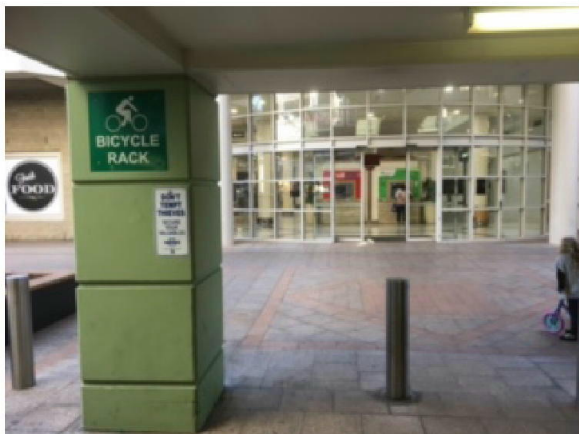
Photograph 1: Centre Entry from Waste Holding Room
