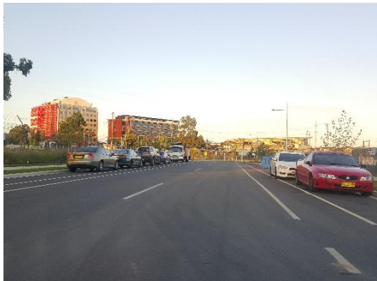
Figure 2.3: Lord Sheffield Circuit (looking west) at the southern end of Aviators Way
