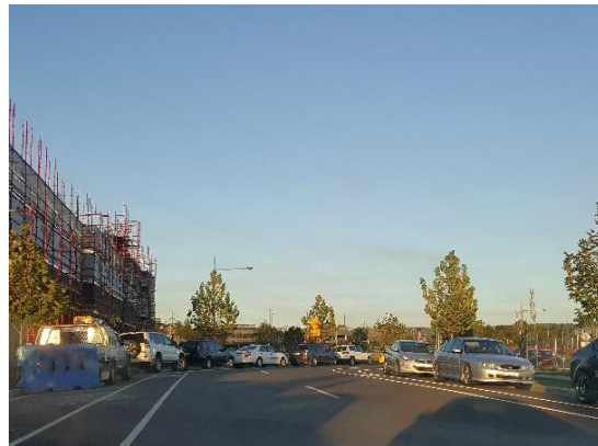
Figure 2.4: Lord Sheffield Circuit (looking west) at the northern end of Aviators Way
