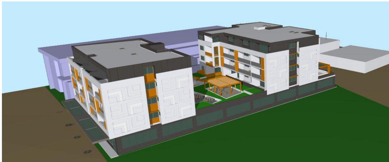
3 WEST COURT YARD
