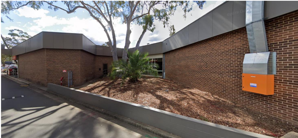
Figure 6. Existing courtyard area (main building) looking north-east
