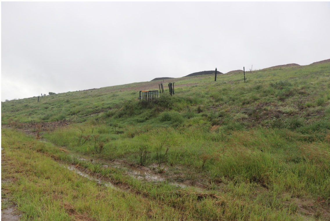
Photograph 13: View of batter on the northern side of the landfill with the landfill gas collection system infrastructure visible. Surface water run-off is collected in spoon drains and diverted to one of two dams on site.
