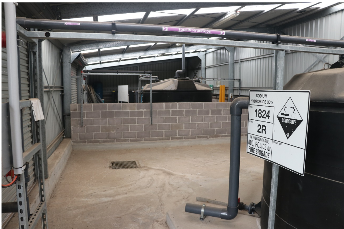
Photograph 8: View of interior of the Leachate Treatment Plant, note that significant staining or deterioration of the concrete slab was not apparent.
