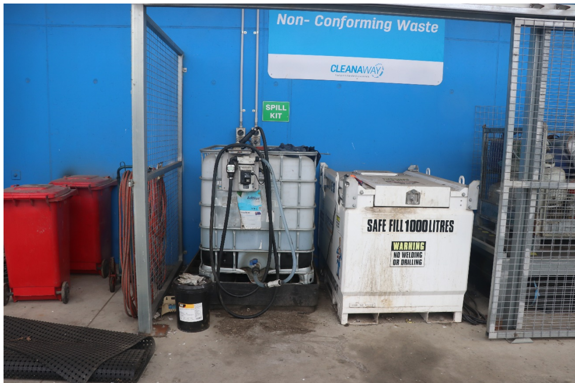
Photograph 5: 1,000L diesel day-tank and diesel exhaust additive (“AdBlue”) in IBC on the eastern exterior of the Transfer Station.
