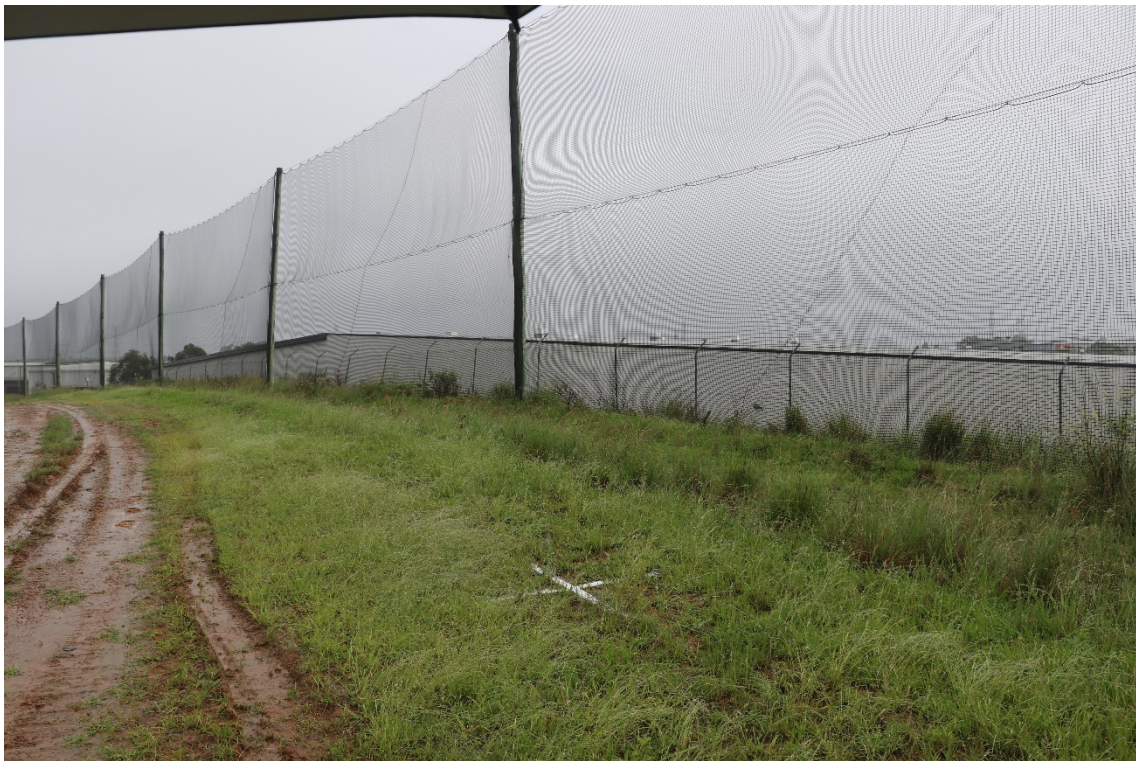
Photograph 17: Permanent litter trap netting at the north eastern corner of the site.
