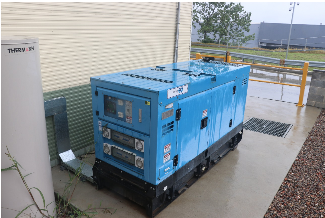
Photograph 2: Back-up generator located at the eastern end of the Administration Building. No concrete staining was observed.
