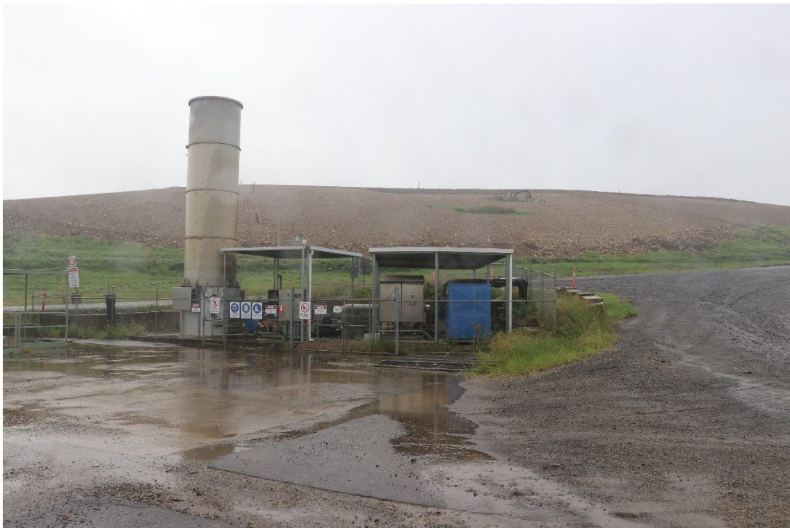
Photograph 14: Landfill gas flare located on the western boundary of Lot 4.
