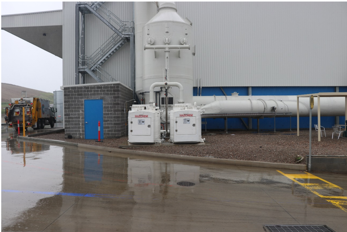
Photograph 3: View of the northern exterior of the Transfer Station with exhaust system. The system uses sodium hypochlorite.
